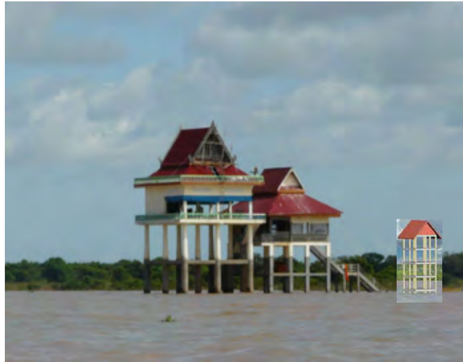
Figure 10.17 Existing Towers located outside of Inundated Forest Area
