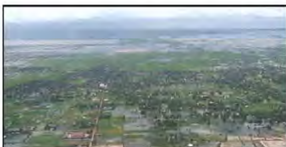
Photo-3: Overview of the candidate WTP site (Upper-side; Tonle Sap Lake, Lower-side; Siem Reap town)
