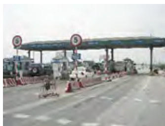
Tollgate on NH.1
