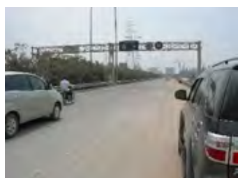
Signs on Ha Noi–Cau Gie
