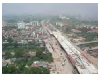
Overview of Ring Road No.3
