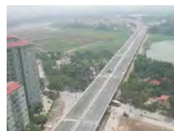
Overview of Ring Road No.3
