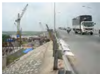
Widening of Bridge on NH.1
