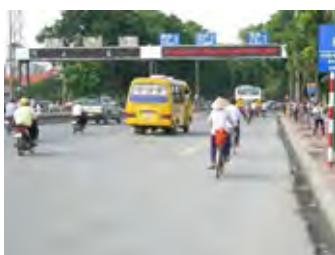
VMS on Ring Road No.3
