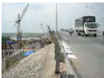
Widening of Bridge on NH.1
