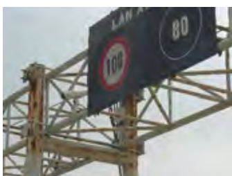
CCTV Camera on Ha Noi-Cau Gie
