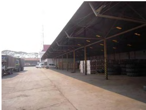
Cargo handling area of existing Thanaleng Truck Terminal
