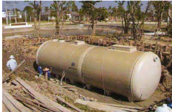
Figure 5.4.5 Sewerage Treatment Facility
