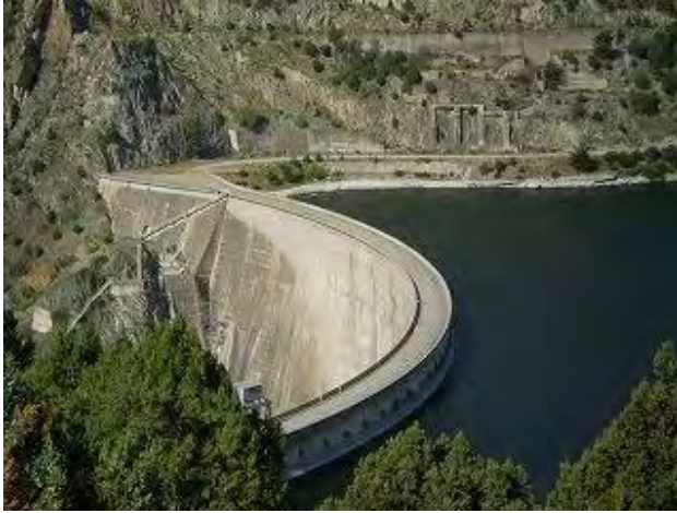
Photo 12 Gökçekaya Dam (as Lower Dam)
