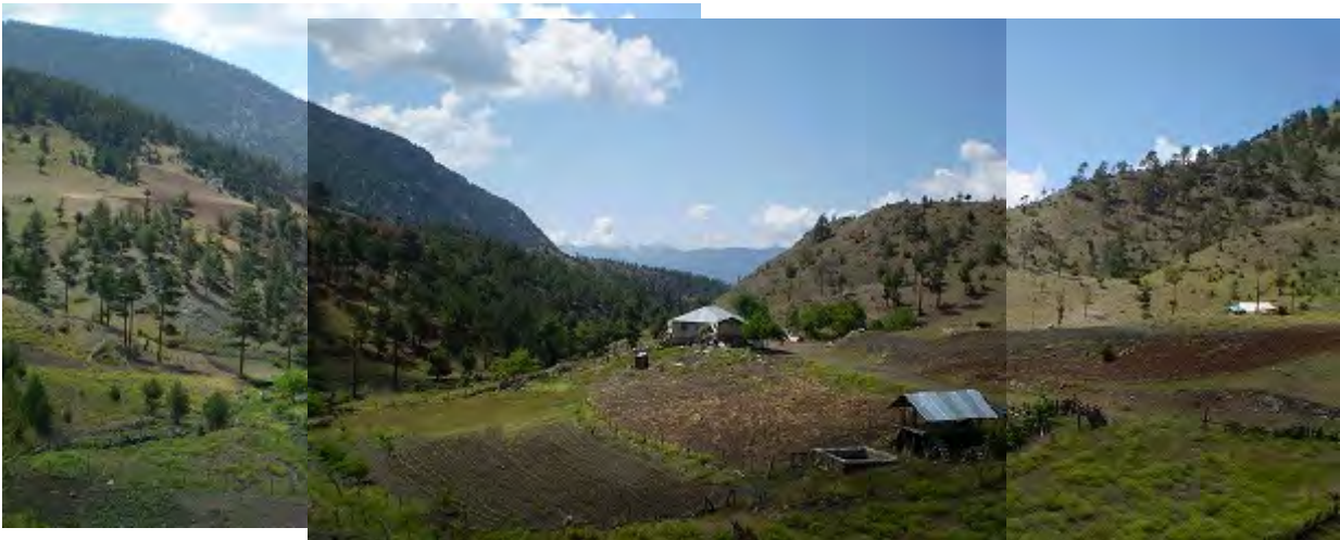
Photo 2 Upper dam site, viewing from the upstream
