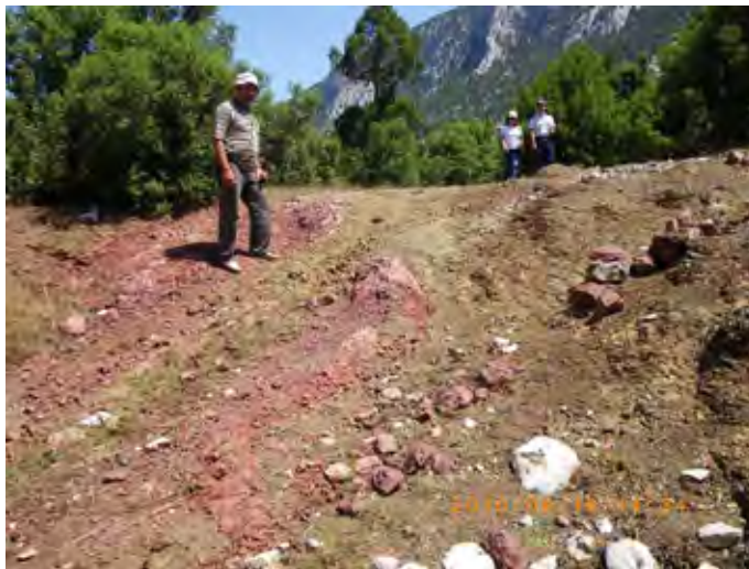
Ophiolitic mélangé of Kirkdirek formation (KKm) distributes at the right bank of the river, and is weathered from moderately to highly. The rock is easily crushable by hammer.
