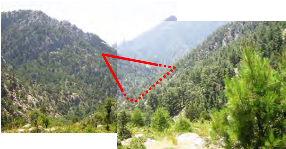
Photo 2 The upper dam site, viewing from the upstream
