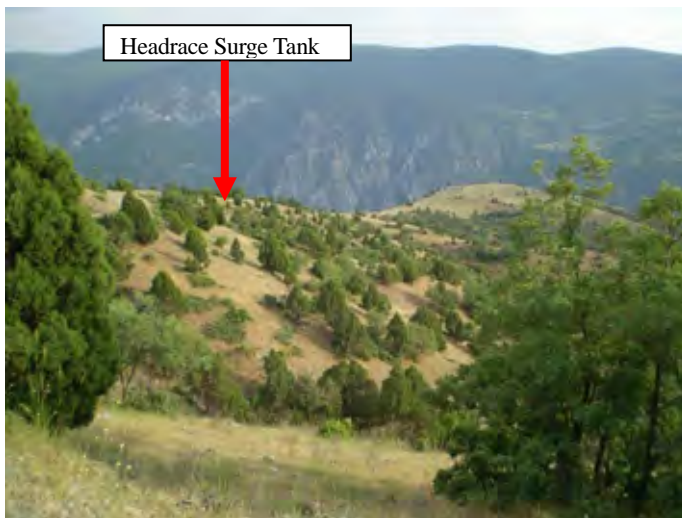
Photo 6 Waterway route and Headrace Surge Tank site
