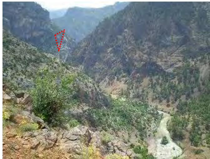
Photo 5 Original lower dam site, viewing from the left bank of upstream.
