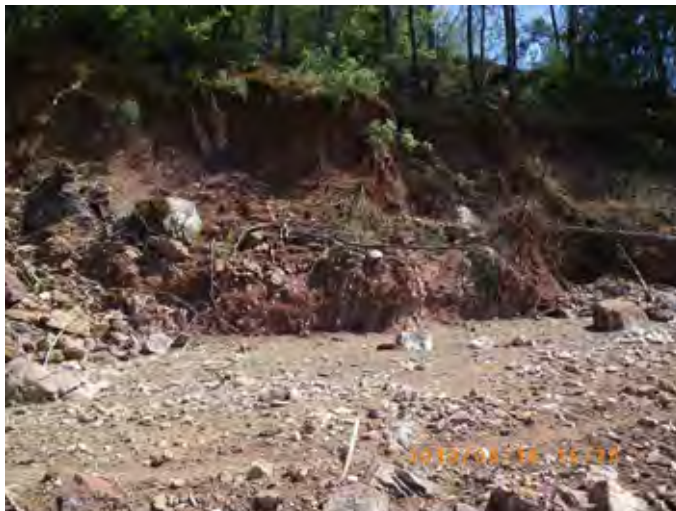
Outcrops of chart eroded by wave Photo 9 Tailrace and Outlet site
