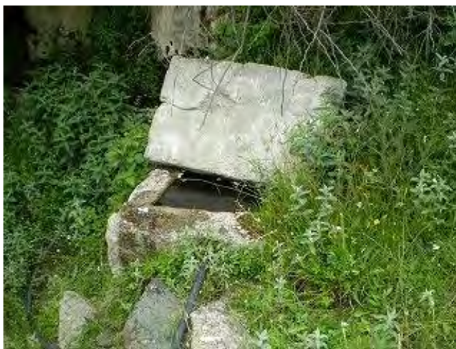
Photo 9 Water tank on the right bank of the upper dam site
