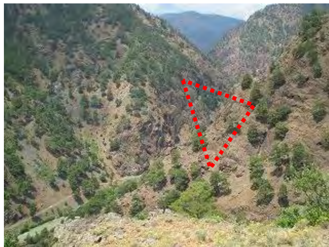
Photo 6 Alternative lower dam site, viewing from left bank of downstream.
