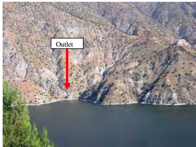
Photo 9 Outlet site, viewing from the left bank
