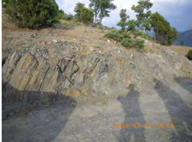
Photo 7 Hard metamorphic rock cropped out along the waterway route
