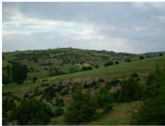
Photo 2 Upper reservoir, viewing from the downstream
