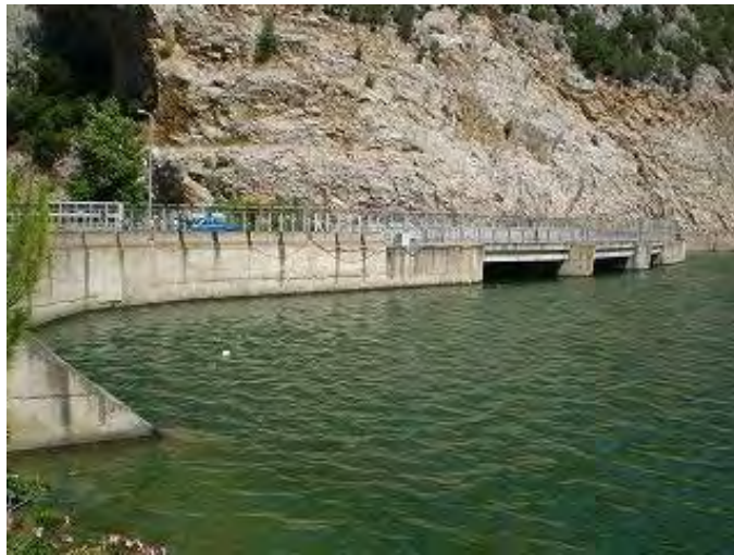
Photo 8 Existing Karacaoren II dam as the lower reservoir
