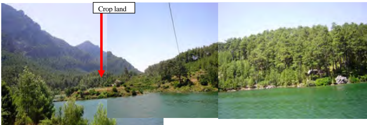
The original outlet site is located at a flat terrace used for farm which height is about 3 meter from the HWL of the reservoir and the slope is gentle with approximately 20 degrees.
