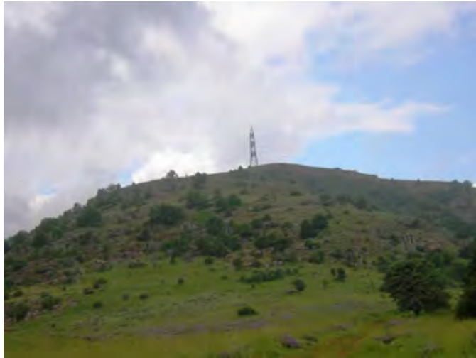
Photo 4 Transmission steel tower at the upstream of the upper reservoir
