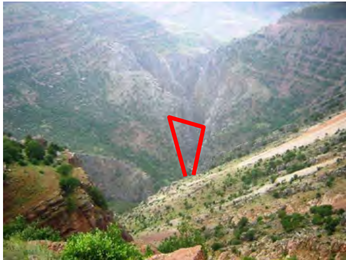
Photo 5 Lower dam site viewing from right bank
