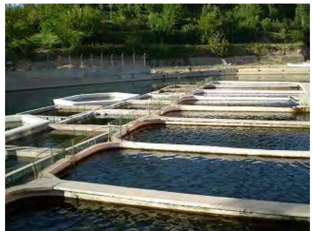
Photo-21 Fish ponds utilizing Leakage Water
