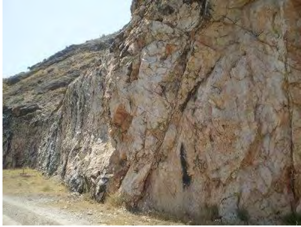
Photo-10 Limestone at Left Bank
