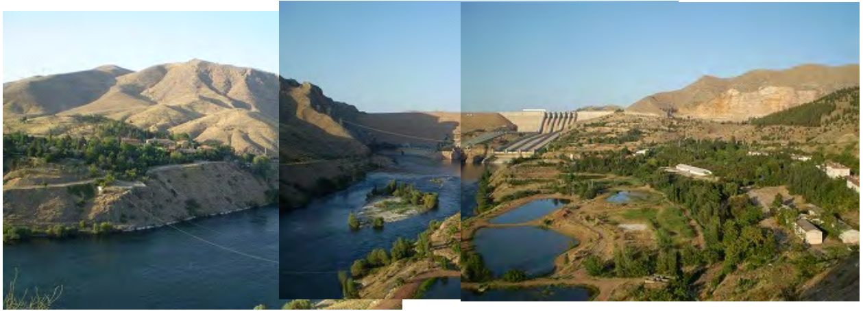
Photo-1 Keban Dam, view from downstream.
