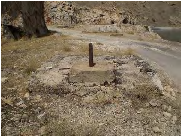
Photo-12 Grouting Pipe
