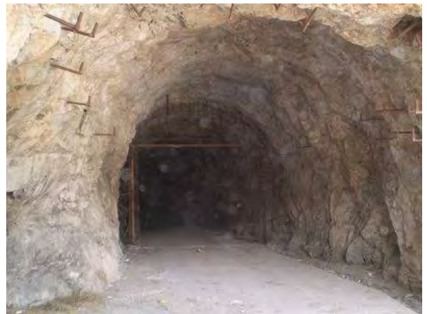
Photo-13 Limb Grouting Tunnel
