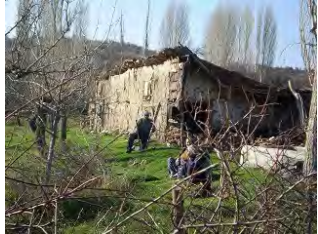
Photo 5.44 House to be resettled (Second House)
