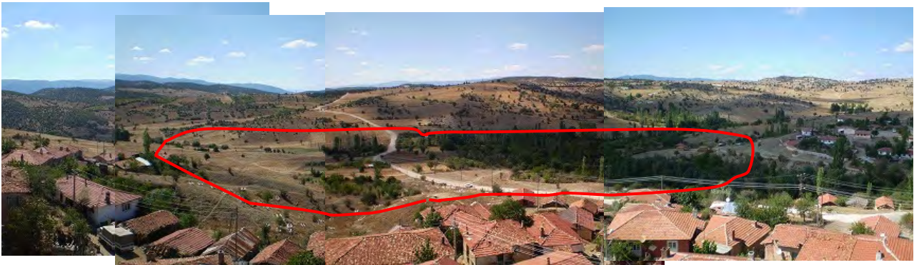
Photo 5.39 Upper Reservoir Site (viewing from left bank)
