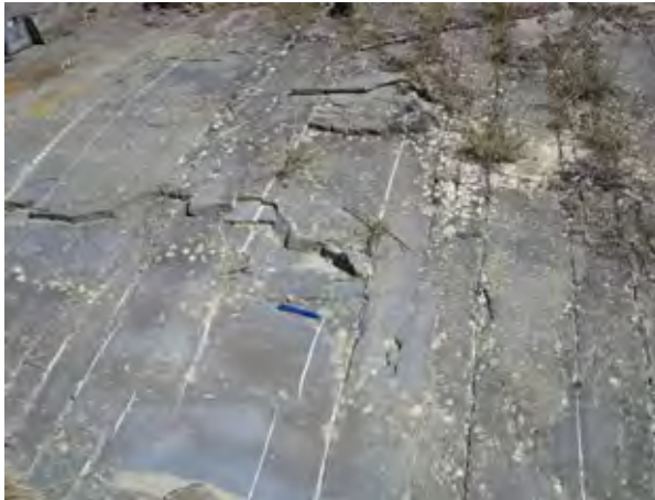
Photo 5.9 Calcite veins filled in joints of sandstone
