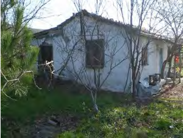
Photo 5.43 House to be resettled (Second House)
