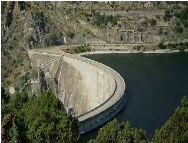
Photo 5.37 Gökçekaya Dam (as Lower Dam)
