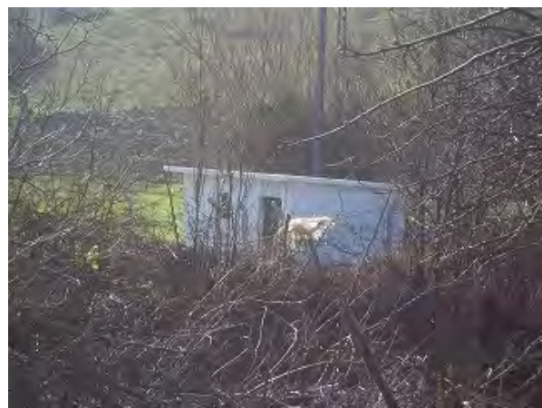
Photo 5.36 New Pumping-up Facility
