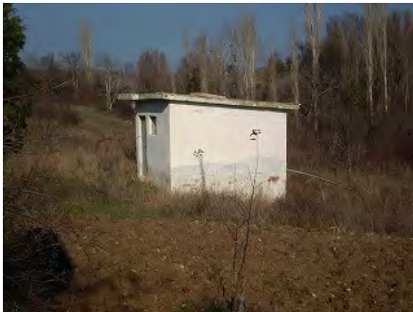
Photo 5.35 Existing Pumping-up Facility
