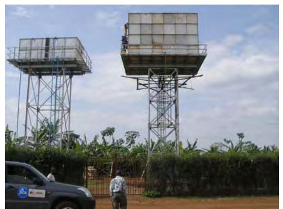
Elevated Tank of RWASCO (Former ELECTROGAZ)
