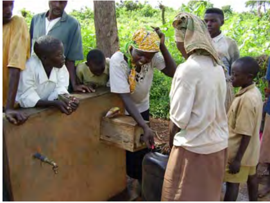
Public Tap Stand of Piped Water Scheme
