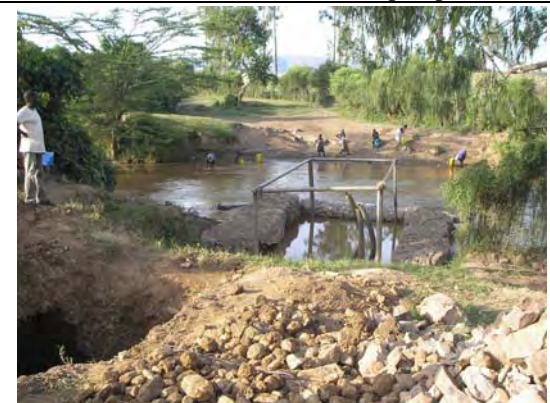
Muvumba River Intake Facility
