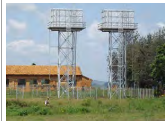
Elevated Water Storage Tank
