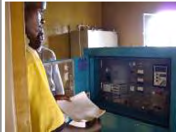
Generator Inspection by Pump Technician
