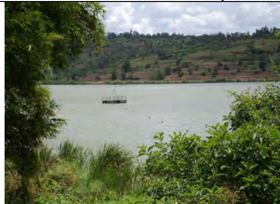
Intake Point of Lake Cyohoha Sud to supply water to Bugesera District
