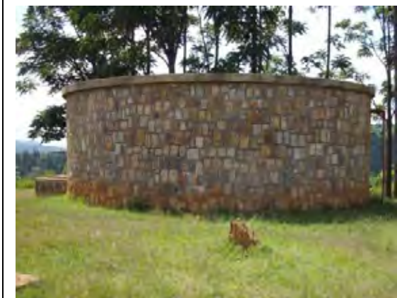
Locally Constructed Water Storage Tank
