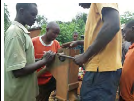
Repairing Handpump by WUA Technician
