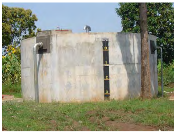
Water Tank of Japanese Grant Aid Project
