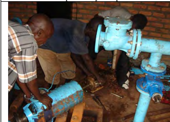
Repairing Transmission Pump
