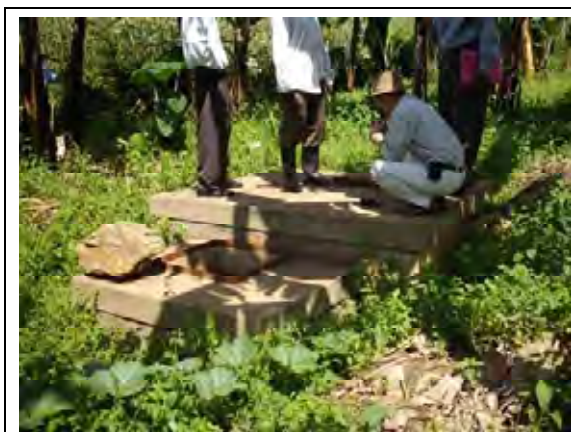
Intake Facility Survey
