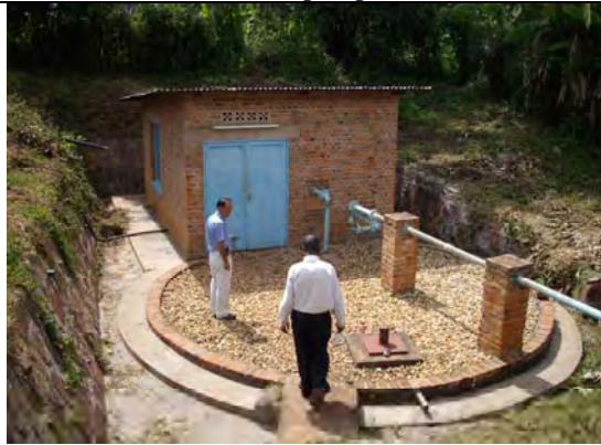
Spring Intake Facility
