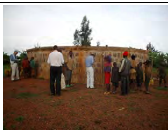
Water Storage Tank Survey
