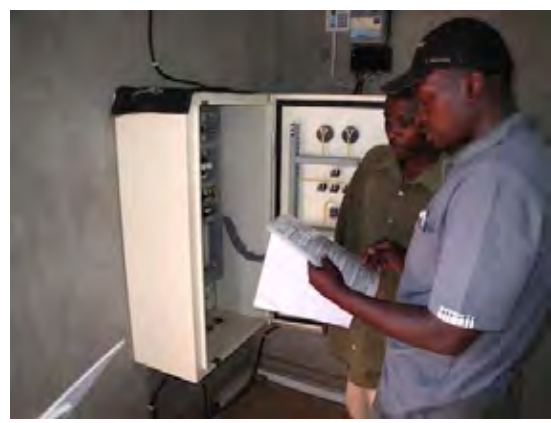
Control Panel Inspection by Pump Operator
