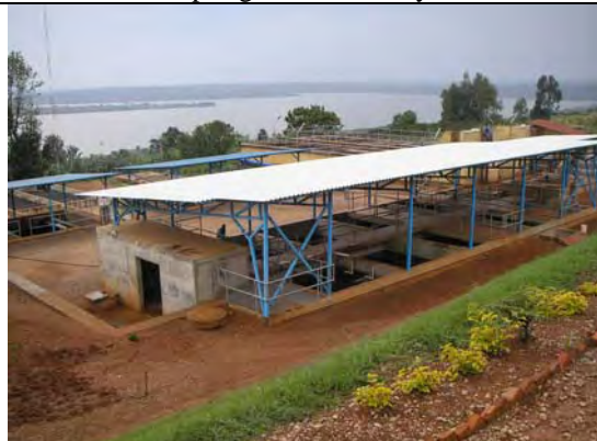
Karege Treatment Plant with Lake Mugesera water source in back
