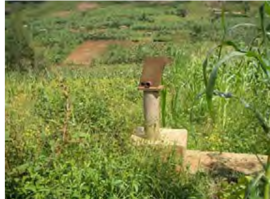
Abandoned Broke n Handpump
