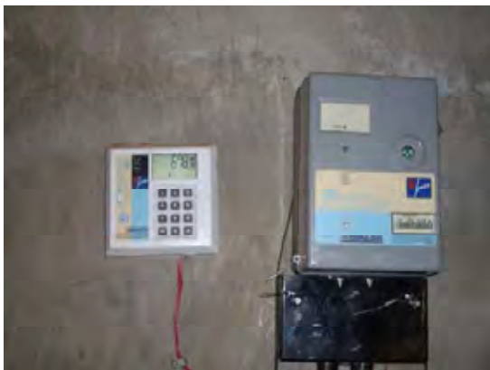
Prepaid device for commercial power
