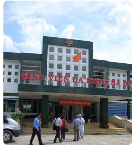
Sa Dec Inter-district General Hospital
