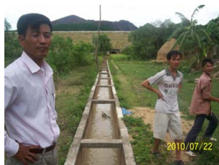
Main Concrete Flume Canal
