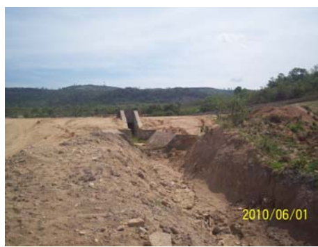
Destructed Canal Caused by Floods
