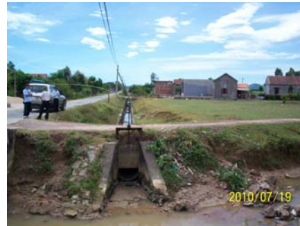
Division Works to SPL Canal
