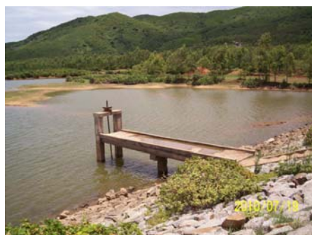
North Intake Facility of Dam
