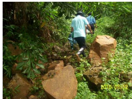
Destructed Canal Caused by Falling Rocks
