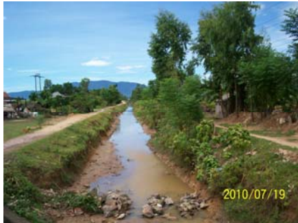
Earth Lining Canal Located in the Upstream of SPL Canal
