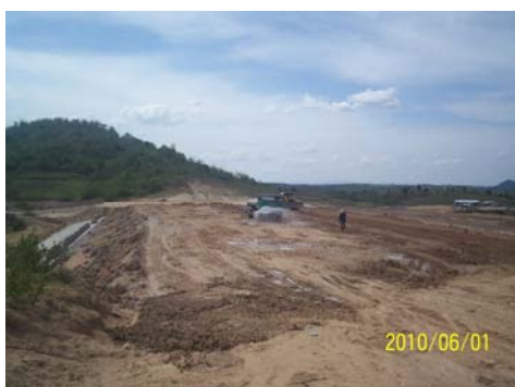
Dam under Construction
