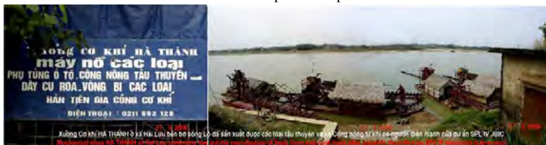
Figure 6.2-7 Mechanical Shop on Lo River Bank, Engineering Ferries Ready to be Handed Over to Customers
