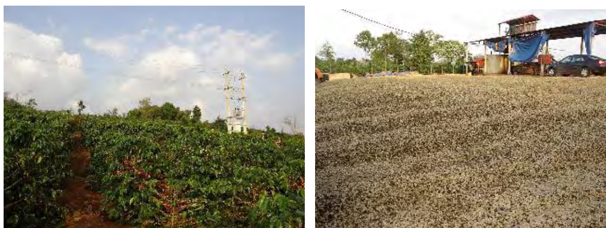
Figure 6.2-2 Coffee Field in Doa Cu Hamlet and its Distribution Transformer, Coffee Preparation Shop Energized by SPL IV
