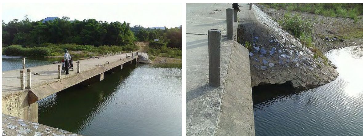
Figure 4.3-6 Conditions of Damaged Safety Posts and Damaged Slope Protection (Left: Damaged Safety Posts, Right: Damaged Slope Protection)
