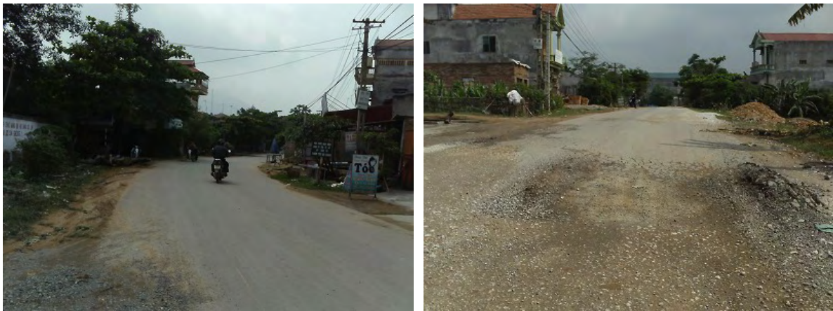
Figure 4.3-18 General View and Rutting Section near Km 1+150 (Left: General View, Right: Deep Rutting Section)
