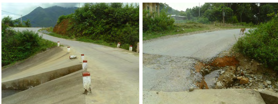
Figure 4.3-17 Spillway Conditions near Km 6+500
