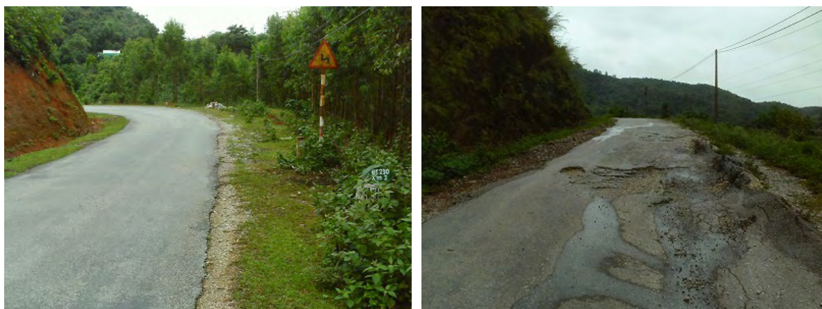
Figure 4.3-13 General View and Deep Rutting Section near Km 2+800
