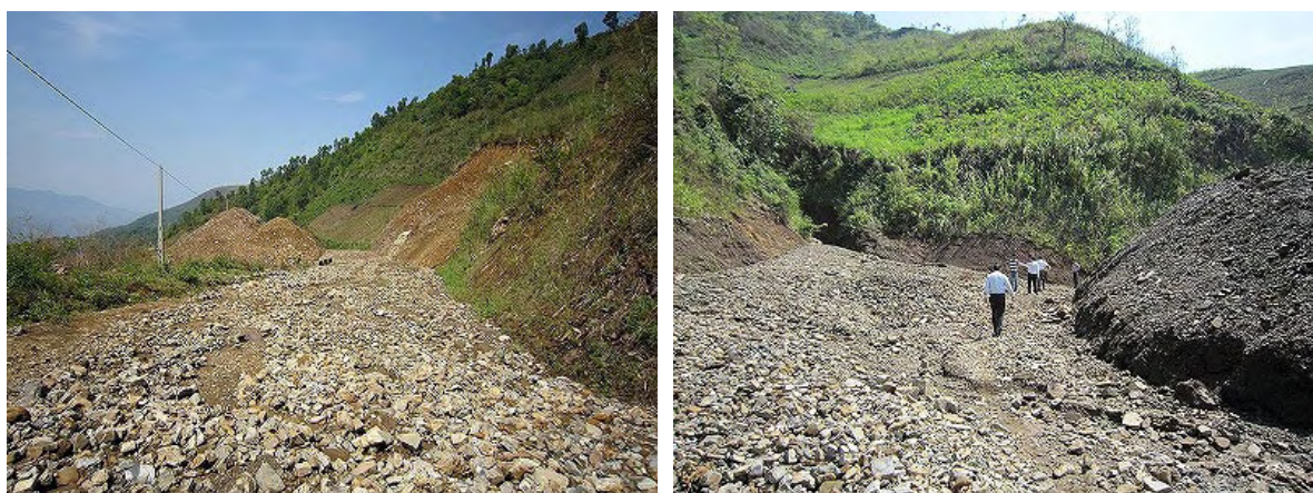
Figure 4.3-4 Condition of Buried Road Section at Km 16
