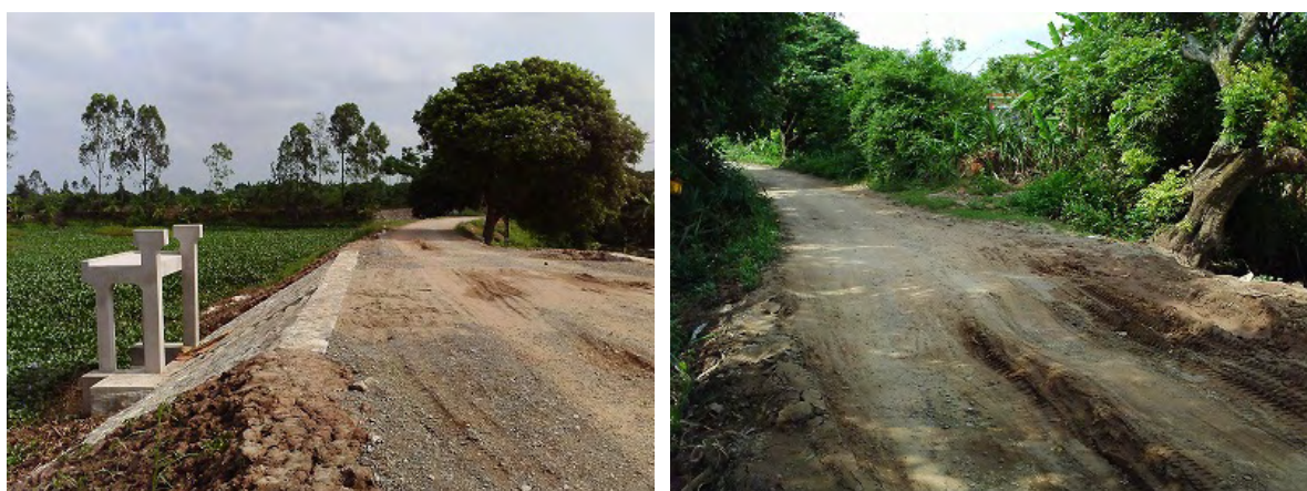
Figure 4.3-20 General View and Rutting near Km 4+000
