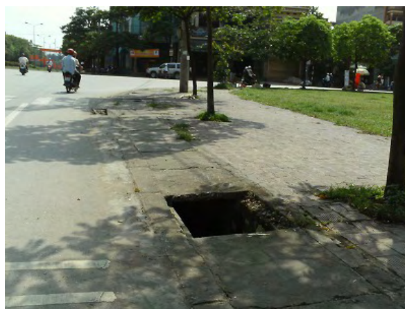
Figure 4.3-14 Side Ditch without Cover
