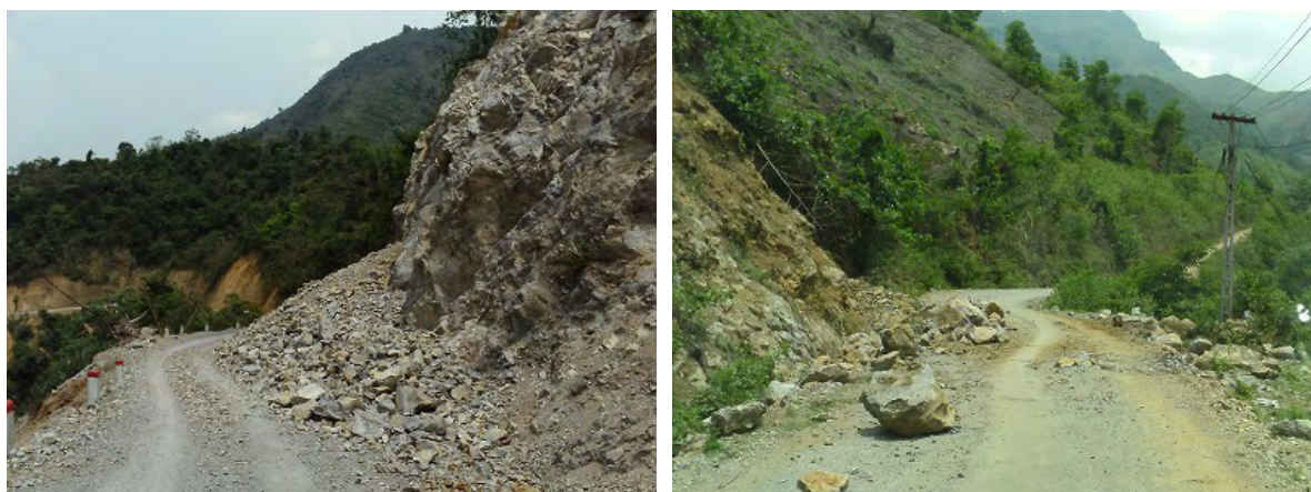
Figure 4.3-5 Condition of Ripped Rock Section at Km 75+100, Fallen Rocks at Km 80+700 (Left: Km 75+100, Right: Km 80+700)
