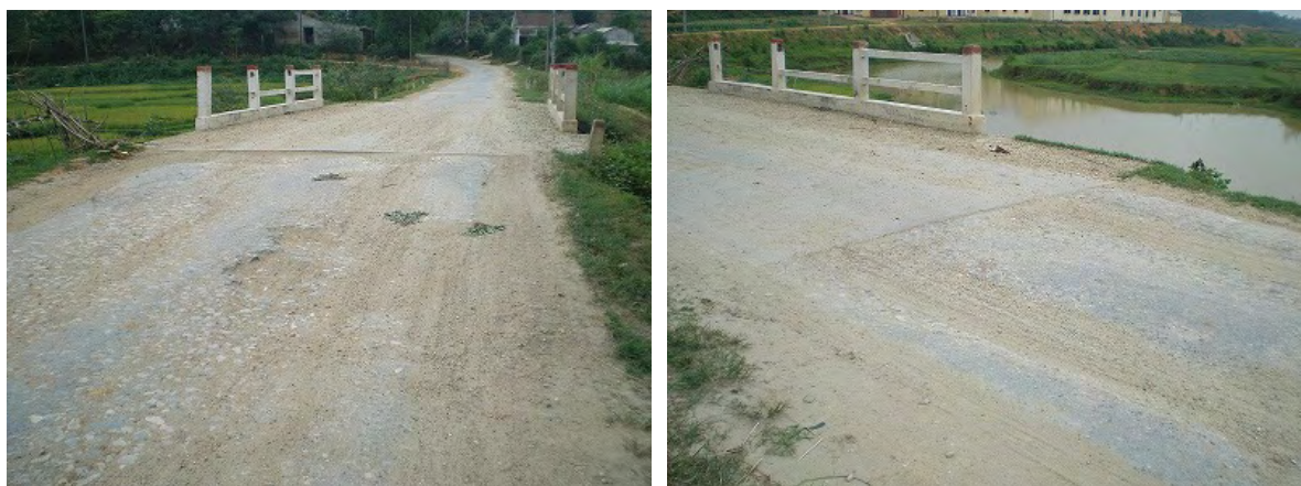
Figure 4.3-15 Damaged Guardrail Beam at a Bridge near Km 1+500
