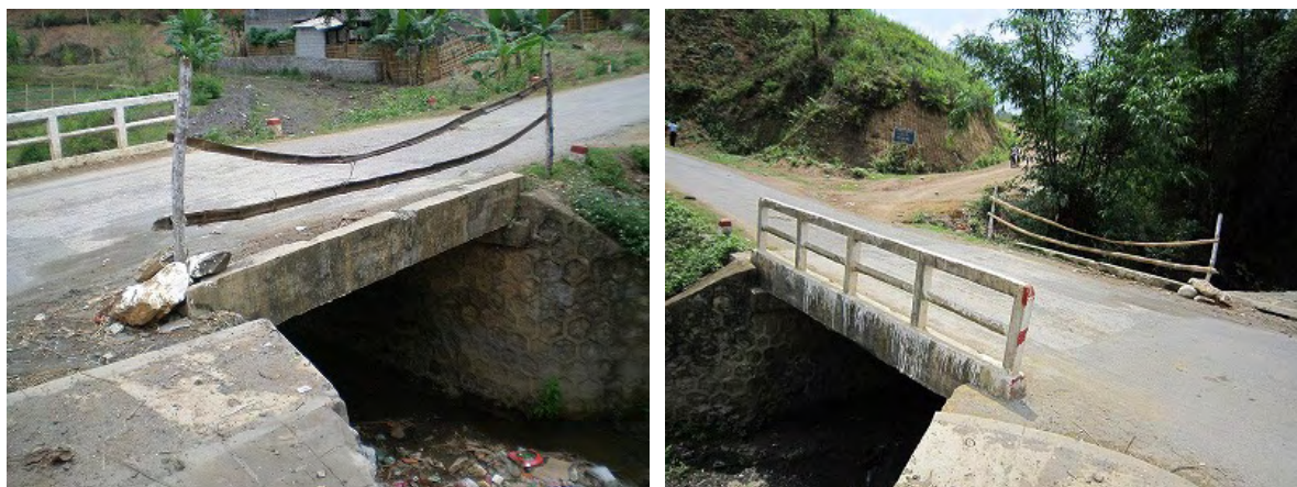
Figure 4.3-10 Damaged Handrail of Bridge at Km 12+700
