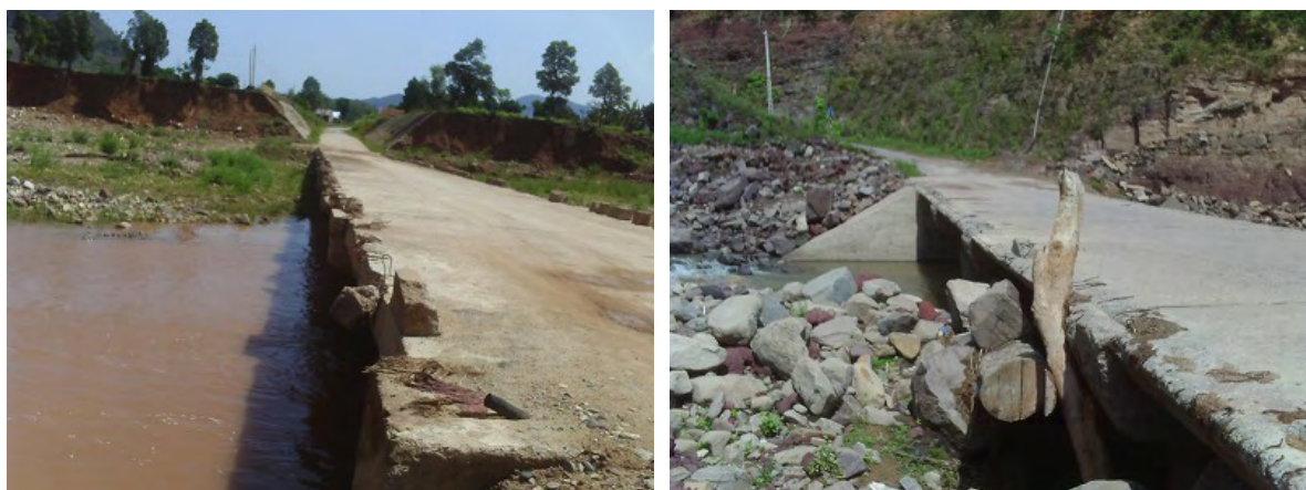
Figure 4.3-7 Damaged Safety Posts and Surface at Km 1+200, Blocked by Obstacles at Km 4+450 (Left: Km 1+200, Right: Km 4+450)
