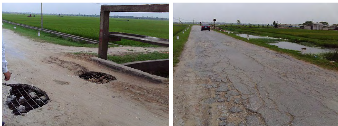
Figure 4.3-19 Damaged Deck Slab at Quan Thu Bridge, Road Surface of the Backside of Abutment
