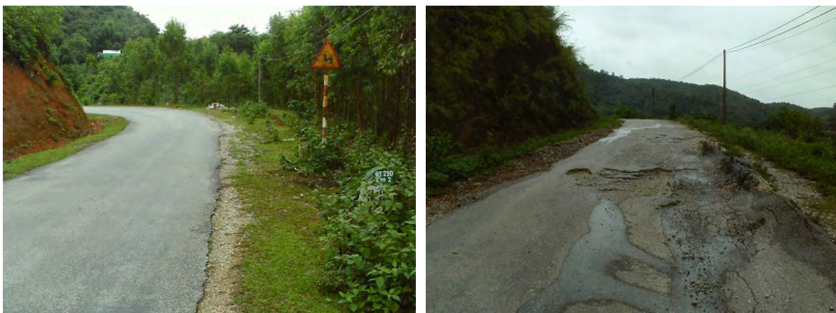
Figure 4.1-14 General View and Deep Rutting Section at near Km 2+800
