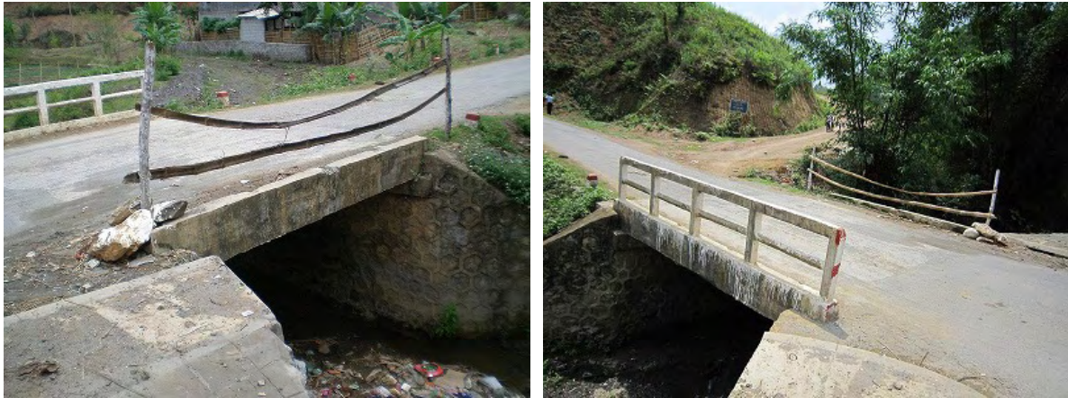
Figure 4.1-11 Damaged Handrail of Bridge at Km 12+700
