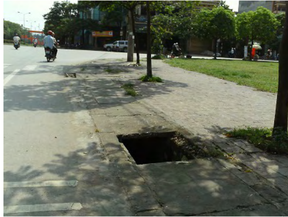
Figure 4.1-15 Side Ditch without Cover
