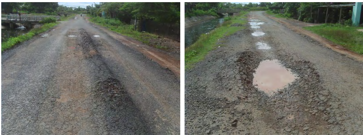
Figure 4.1-23 Damaged Road Surface near Km 0+700, Km 0+850 (Left: Km 0+700, Right: Km 0+850)
