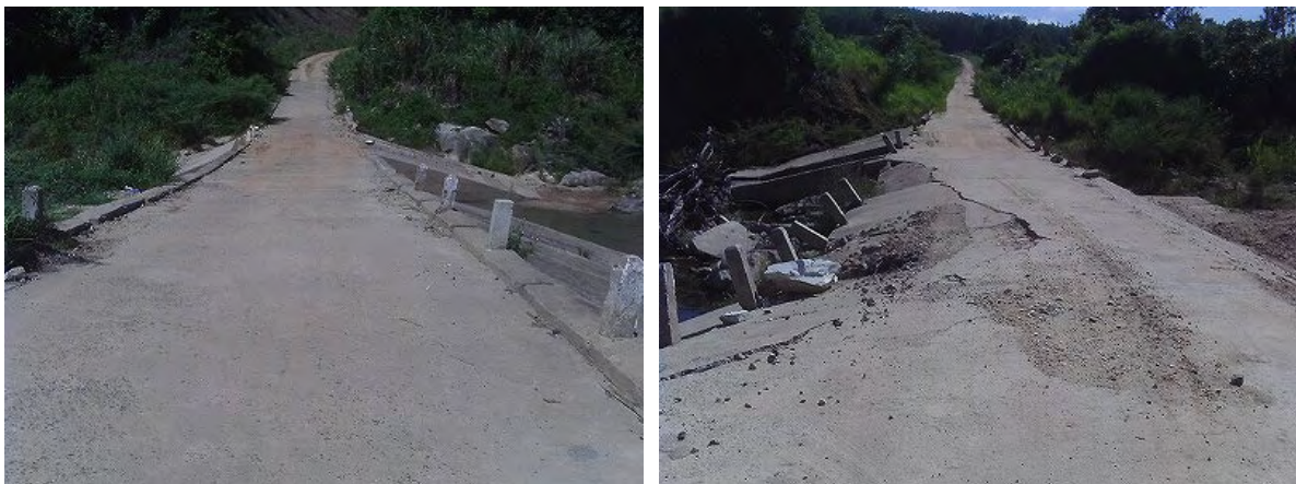
Figure 4.1-9 Overview of the Section at Km10+800, Damaged Spilway at Km10+850 (Left: Km 1+200, Right: Km 4+450)
