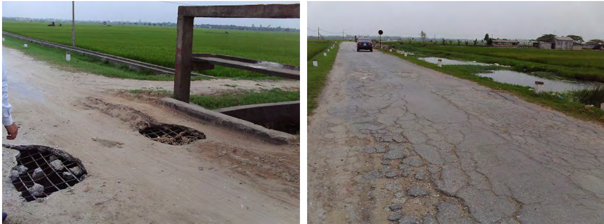
Figure 4.1-20 Damaged Deck Slab at Quan Thu Bridge, Road Surface of the Backside of Abutment
