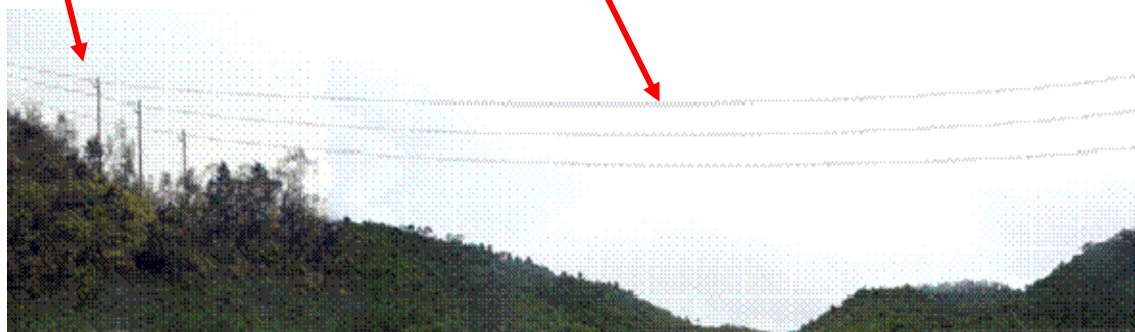
Figure 4.2-10 Long Span Medium Voltage Line (Tuyen Quang Province, Yen Son District)
