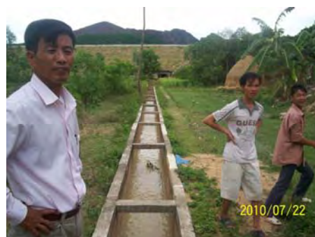
Main Concrete Flume Canal
