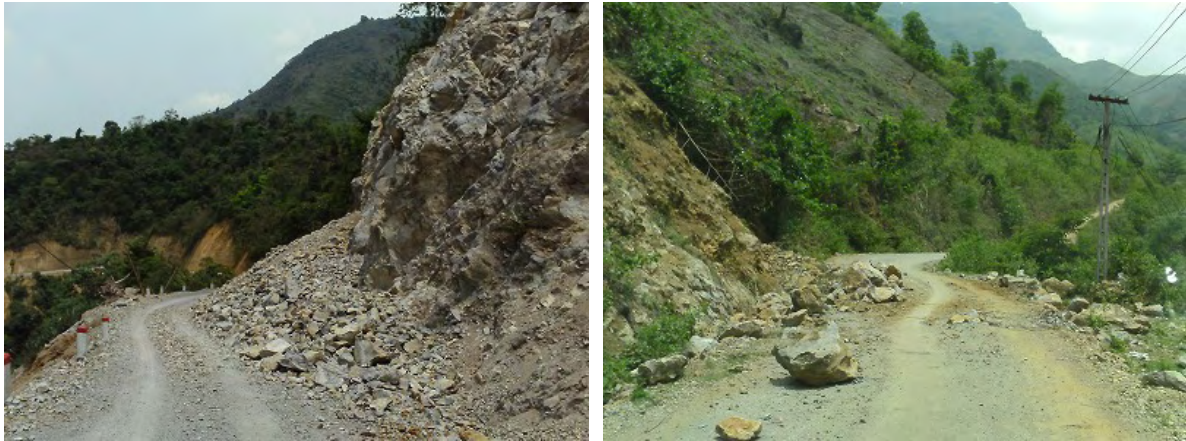
Figure 4.1-6 Condition of Ripped Rock Section at Km 75+100, Fallen Rocks at Km 80+700 (Left: Km 75+100, Right: Km 80+700)
