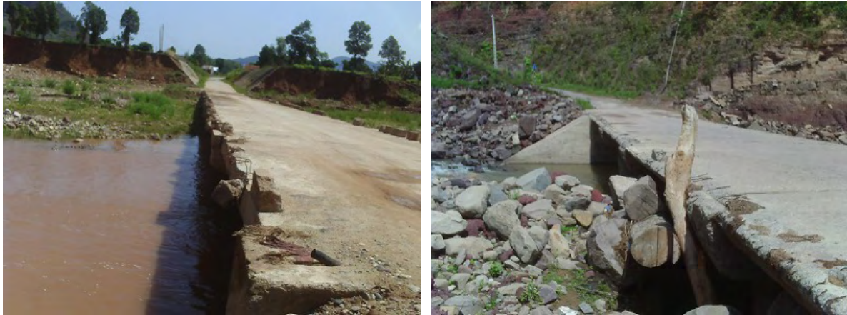
Figure 4.1-8 Damaged Safety Posts and Surface at Km 1+200, Blocked by Obstacles at Km 4+450 (Left: Km 1+200, Right: Km 4+450)
