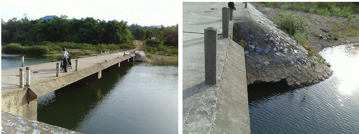
Figure 4.1-7 Conditions of Damaged Safety Posts and Damaged Slope Protection (Left: Damaged Safety Posts, Right: Damaged Slope Protection)
