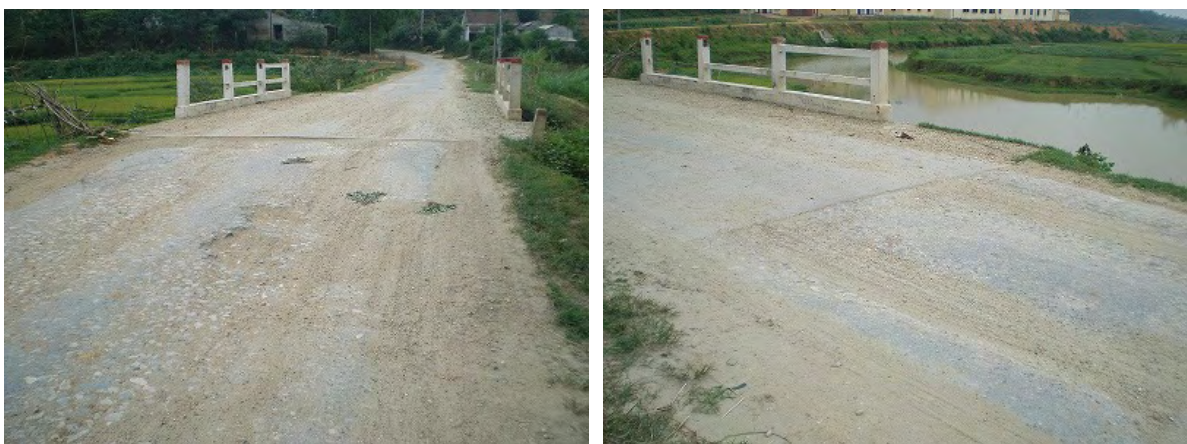
Figure 4.1-16 Damaged Guardrail Beam at a Bridge near Km 1+500
