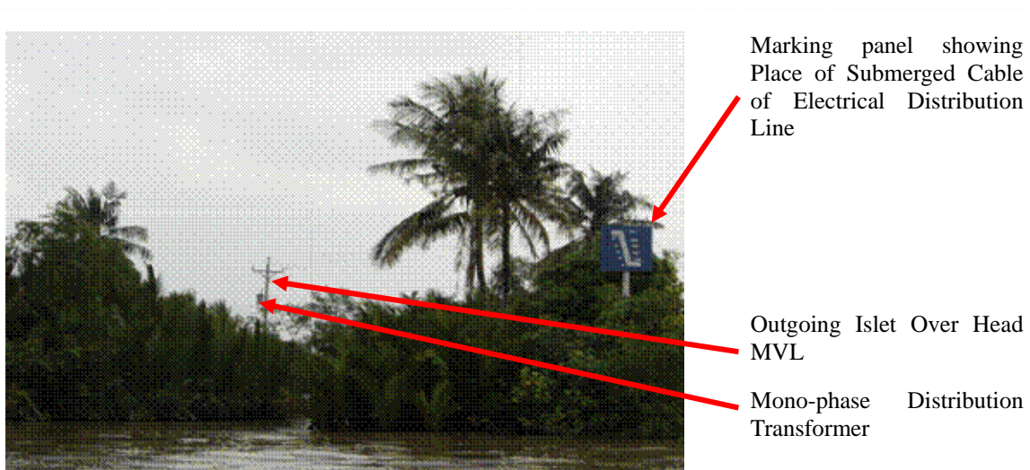
Figure 4.2-8 Submerged Medium Voltage Feeder Cable (Ben Tre Province, Ke Sach District)
