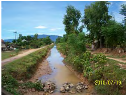
Earth Lining Canal Located in the Upstream of SPL Canal
