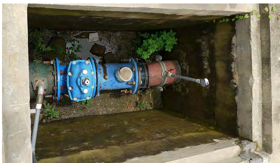
Figure 5.3-3 Condition of Flow Meter Installation
