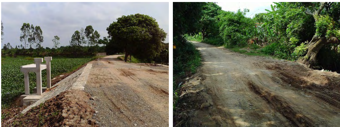
Figure 4.1-21 General View and Rutting near Km 4+000
