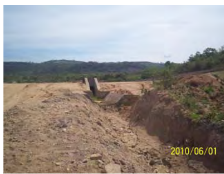
Destructed Canal Caused by Floods
