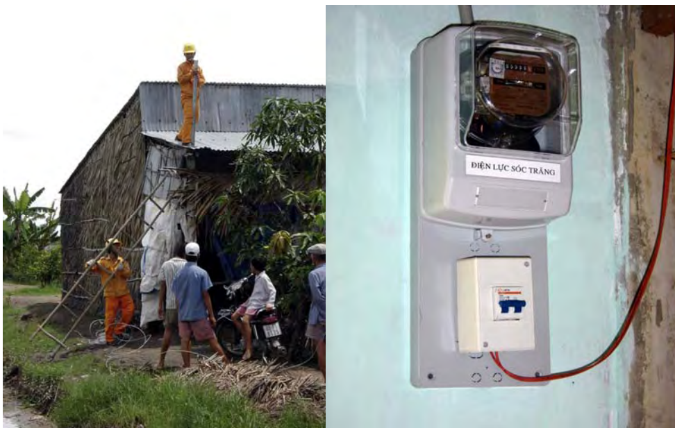
Figure 4.2-6 Electricity Workmen Implementing the Drop Service for Inhabitants' Household in Thanh Phu Commune of My Xuyen District in Soc Trang Province
