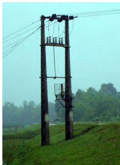
Figure 4.2-4 35 kV Triphases Disconnecter in one of Phu Tho – Vinh Phuc Sub-Projects
