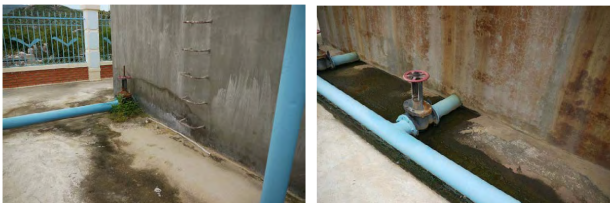
Figure 8.3-1 Examples of Leakage from Reinforced Concrete Structure
