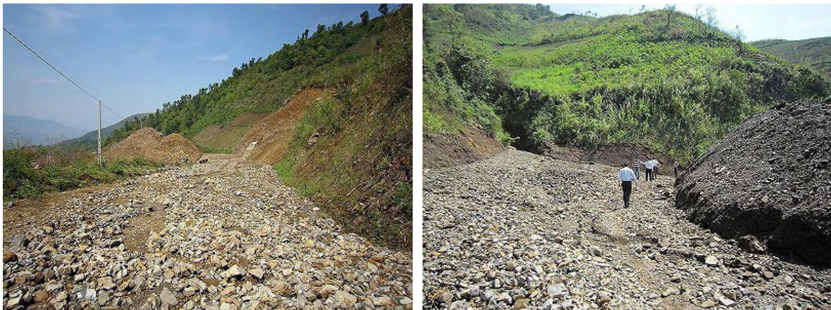
Figure 4.1-5 Condition of Buried Road Section at Km 16
