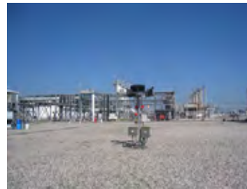
Bibiyana gas plant south area (2009/10/31)
