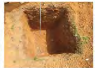
Test pit No.12
