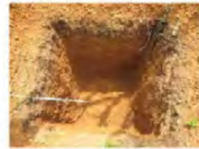
Test pit No.11
