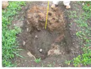
Test pit No.26
