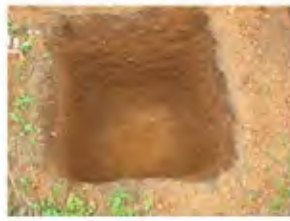
Test pit No.1
