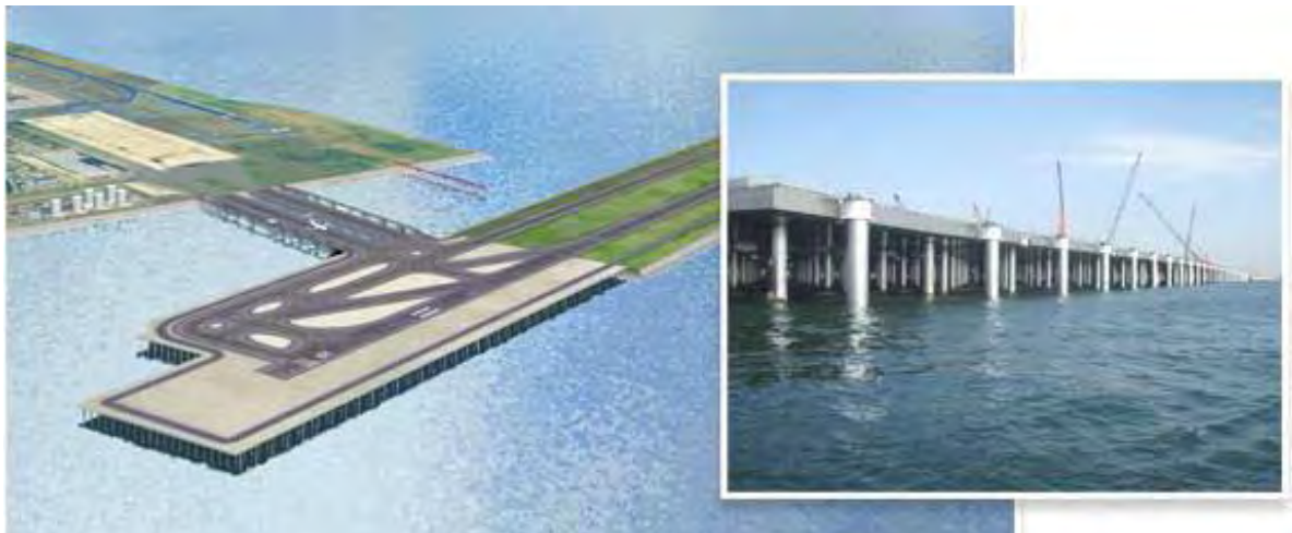
Figure 5.3.53 Example of an On-Pile Structure of Tokyo's Haneda Airport
