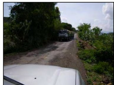
Section of B11 Road where it is difficult for vehicles to pass each other
