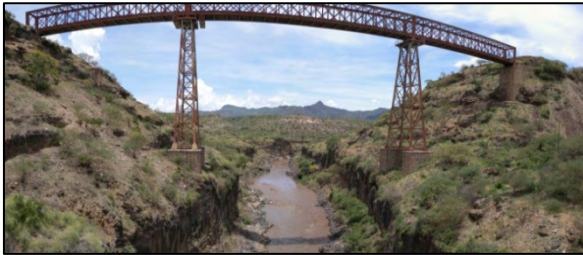
On the upstream side (The foundations of the railway bridge are located above the low-flow channel.)
