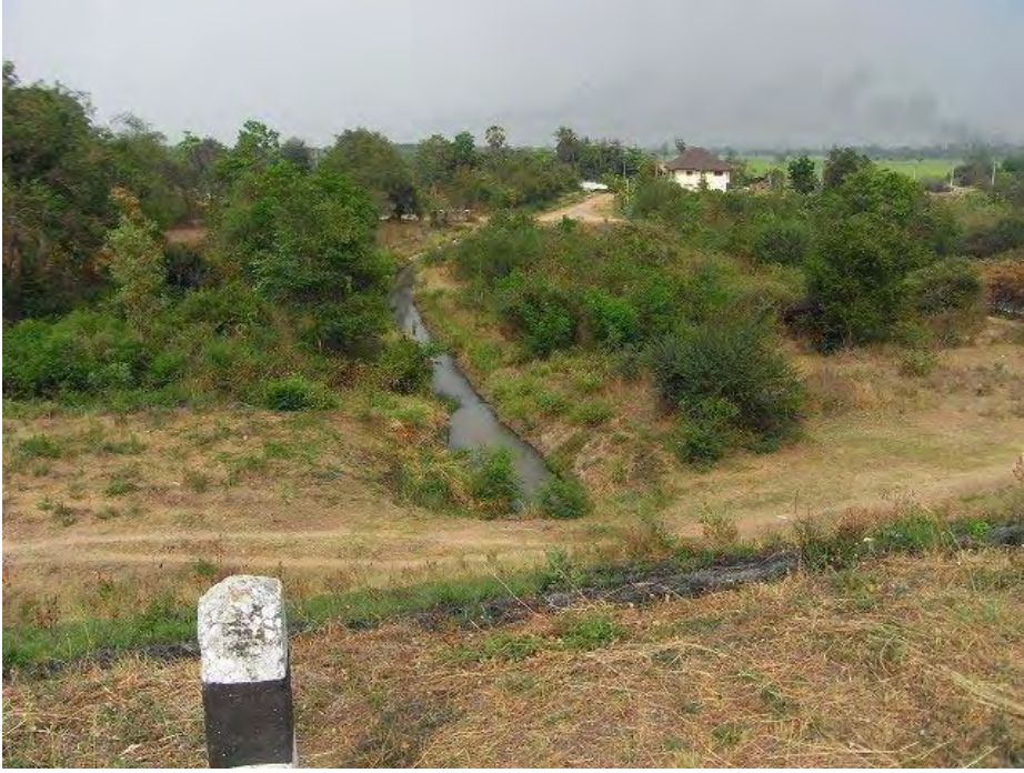
Irrigation Main Canal
