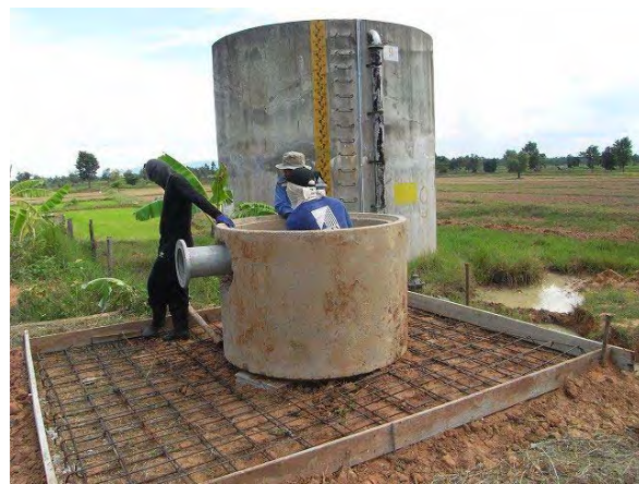
Outlet Tank under repairing
