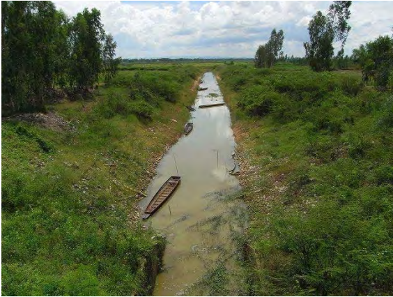
Intake Canal from Ubolrat Reservoir
