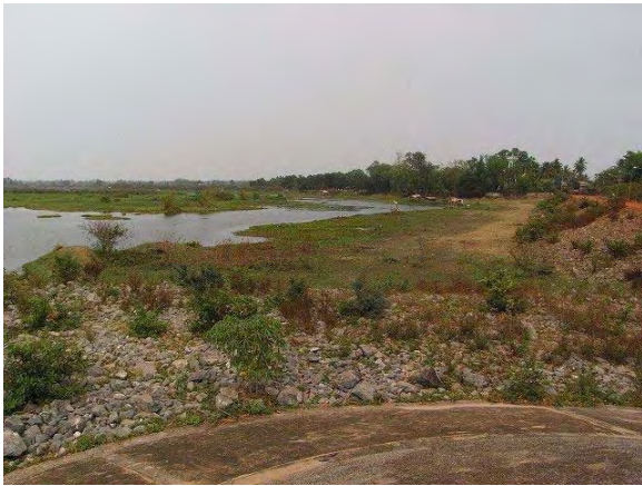
Upstream side of Barrage
