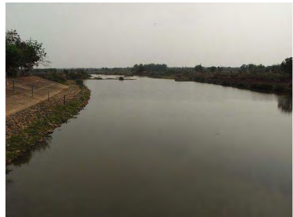
Downstream side of Barrage
