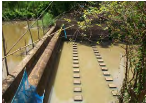
The weir constructed in 1982 (July, 2010)
