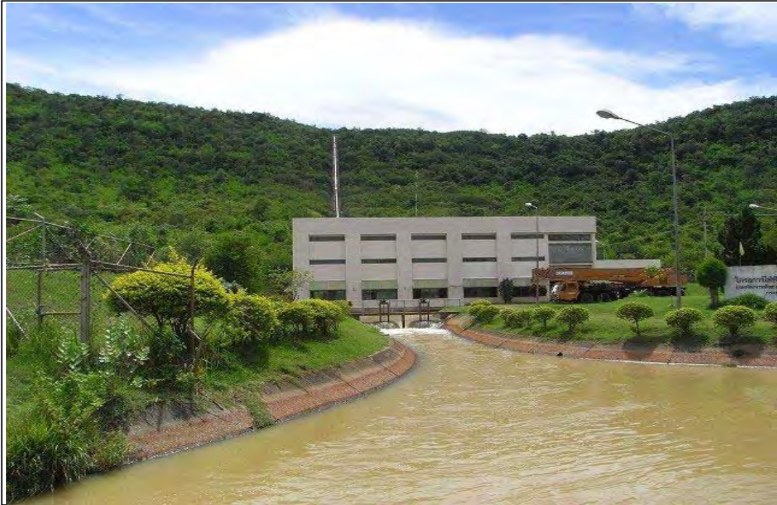
A hydropower plant in the Huai Sam Mo watershed in Chaiya Phum Province. The plant generates electric power by using water of Huai Prathow Dam constructed by DEDP in 1992 and irrigates around 3,000 rai farmlands by trans-basin water diversion.
