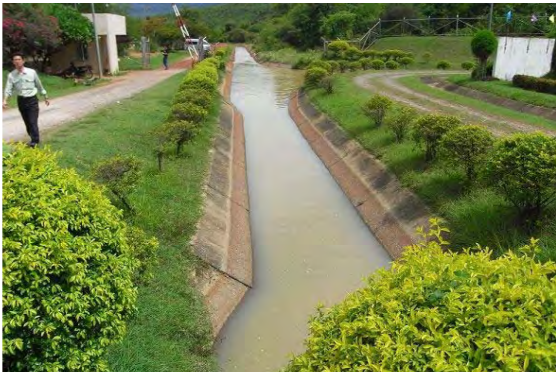
One main canal from the hydro power is shown in the photo above. The estimated discharge of the canal is around 2.5\text{m}^3/\text{s} taking flow of the hydro power. There are three irrigation canals, however, most of water is ineffective outflow. Therefore, DWR diverts ineffective water to six ponds to make use of water as one of watershed management pilot projects.
