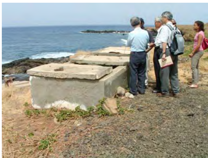
Intake beach well (Praia)
