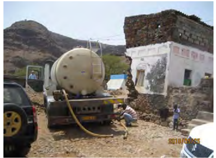
Water Tanker truck & Reservoir (Port Mosquito)
