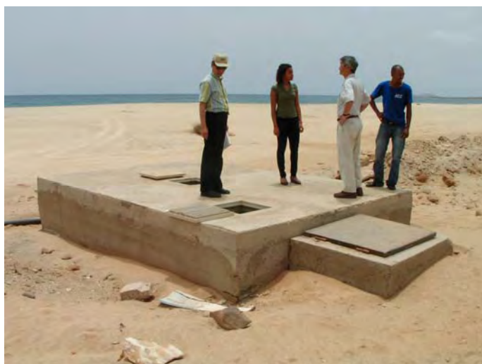
Intake beach well (Sal island)
