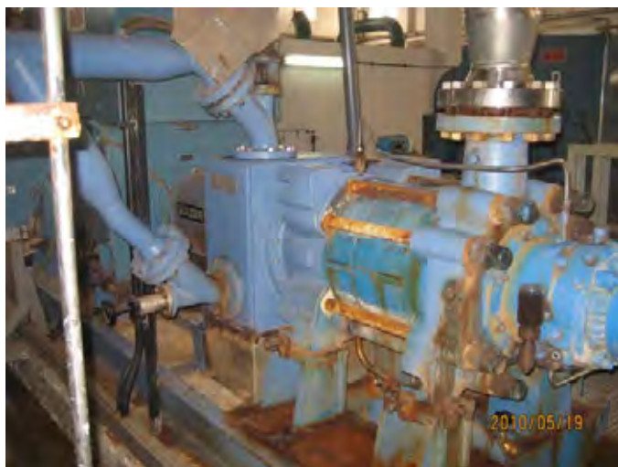
High pressure pump with energy recovery device (Praia)
