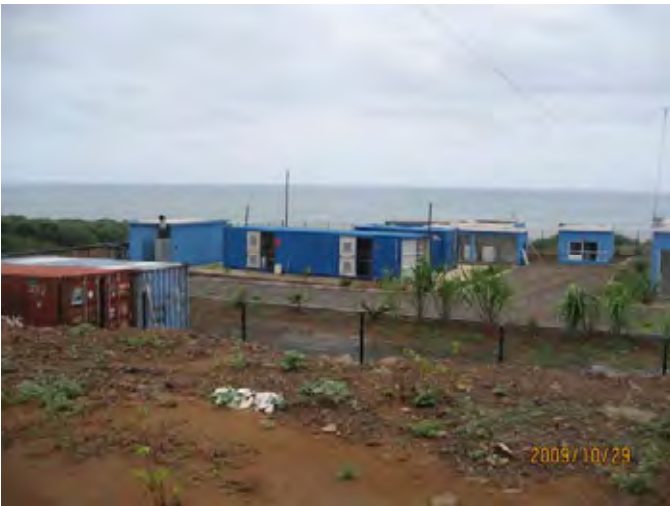
Santa Cruz SWRO plant site
