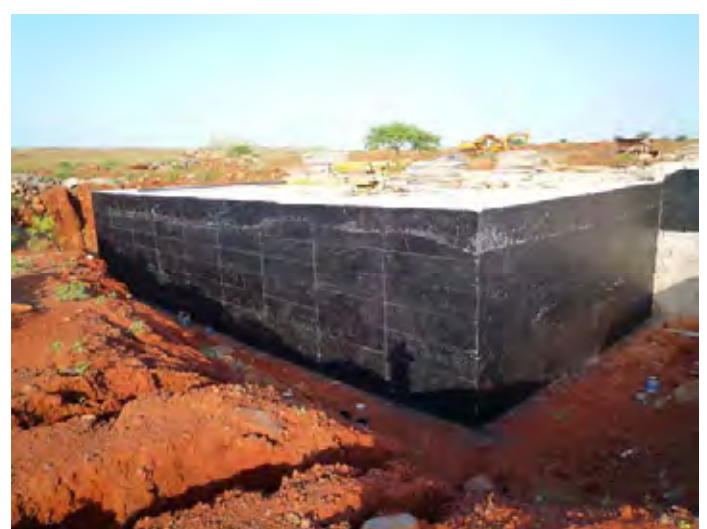
Reservoir under construction (Ribeira Grande)
