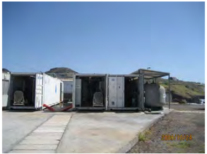
Praia container type SWRO (1,200m 3 /d x 2 units)
