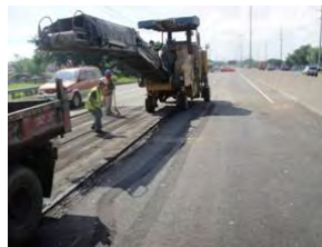
Rotomilling of existing asphalt wearing course
