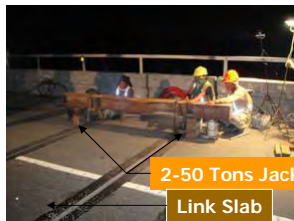
Installation of Carbon Fiber Reinforced Polymer
