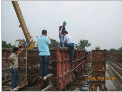
<< Inspection of Precast Girders in Abucay, Bataan
