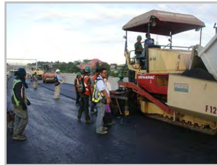
Inspection and Monitoring of >> Stone Mastic Asphalt (SMA) Pavement Laying
