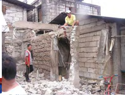
NHA DEMOLITION ACTIVITIES
