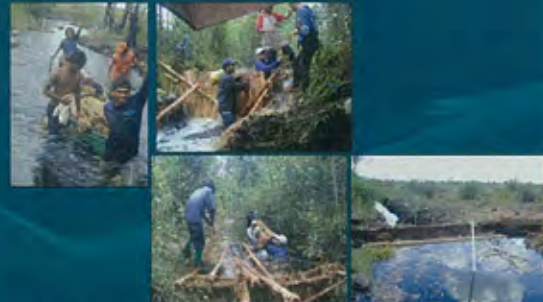
Fig 20. The PUTSK and Local Community establishing dams at the NLPSF
