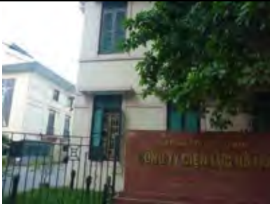
(8) Hanoi Electricity Company
