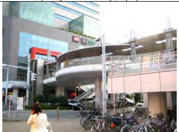
Image of north pedestrian deck to commercial facility (Funabashi Station, Chiba, Japan)
