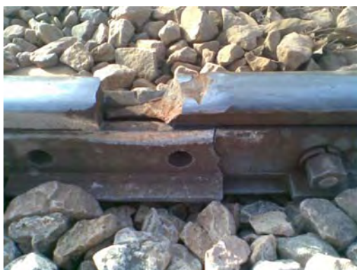
Damaged rail and fishplate without bolts
