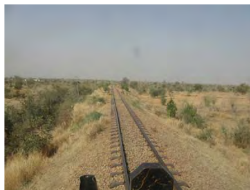
Damaged track due to ballast deficiency
