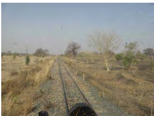
Ballast overflowed onto the slope due damaged embankment shoulder
