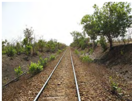
Track between Kotiari and Bala (26 kg/m rail)
