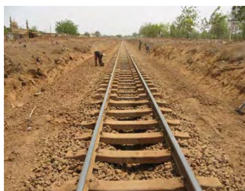
Ballast cleaning and slope stabilization works in the Bobo-Dioulasso direction of Koudougou station
