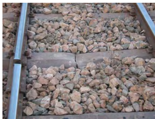
Damaged sleeper and excessive joint gap
