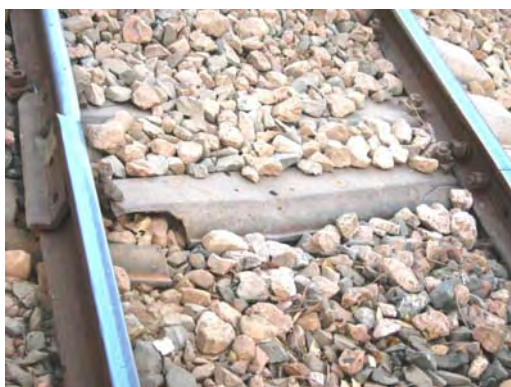
Damaged sleeper and fishplate without bolts
