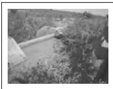
Spillway at 1578m point
