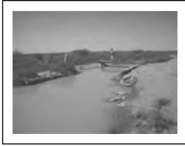
Upper stream of S27 secondary canal diversion
