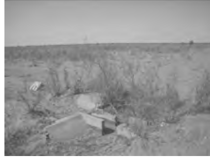
Tertiary canal diversion box
