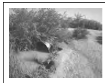
Cross load conduit at about 200m upper stream from spillway
