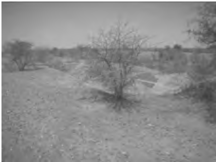
Secondary canal diversion facility
