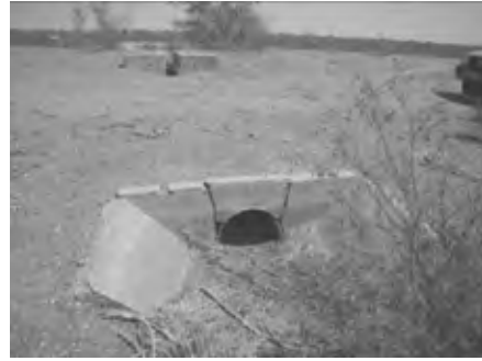
Cross load facility of tertiary canal
