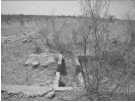
Tertiary canal diversion box
