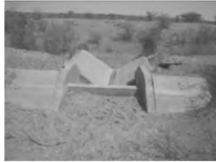
Secondary canal spillway
