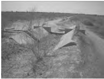
Drop and diversion check gate
