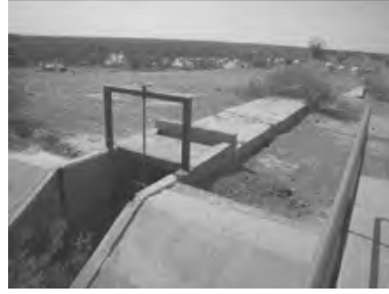
S9 Primary canal diversion facility (Left bank)
