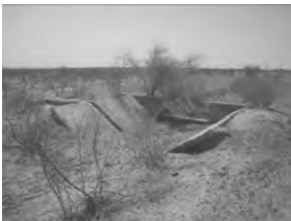
Drop and diversion regulating gate
