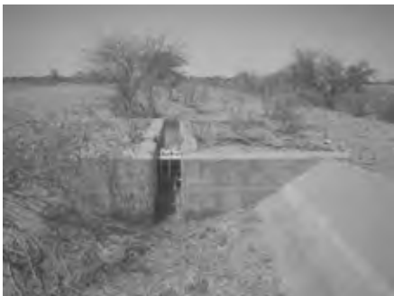
Tertiary canal diversion facility
