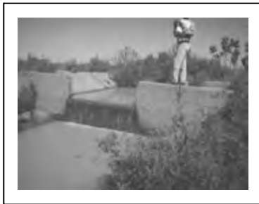
Diversion check gate at 677m point
