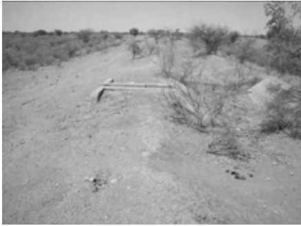
Secondary canal diversion facility
