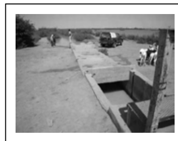
S27 Diversion facility and secondary canal in down stream
