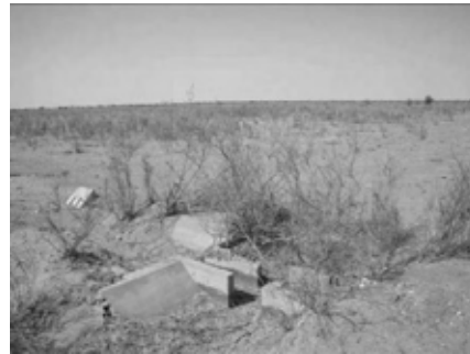
Tertiary canal diversion box
