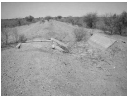
Secondary canal diversion facility
