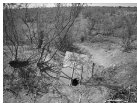
Diversion facility to fourth canal
