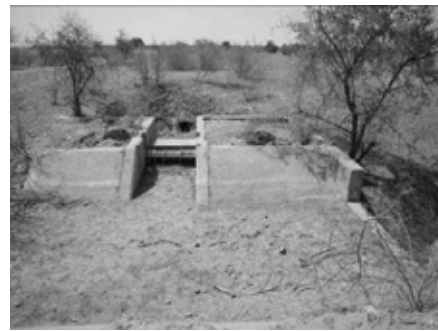
Tertiary canal diversion facility (Module Amasuk)
