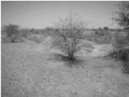
Secondary canal diversion facility
