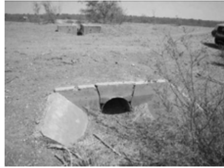
Cross load facility of tertiary canal
