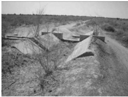
Drop and diversion check gate
