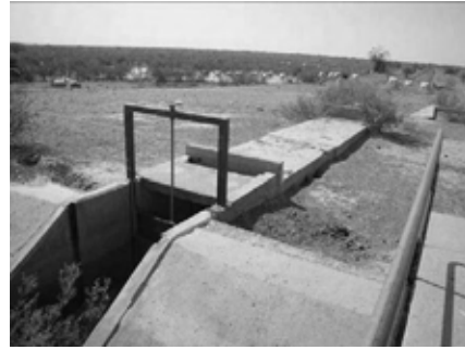
S9 Primary canal diversion facility (Left bank)
