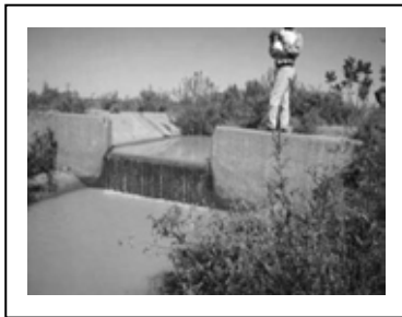
Diversion check gate at 677m point
