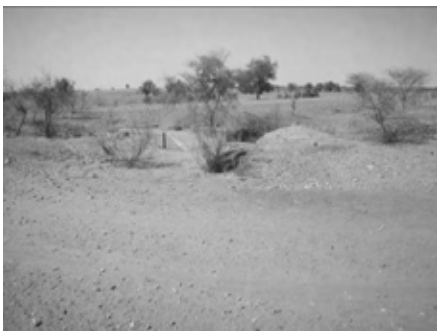
Diversion check gate
