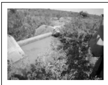
Spillway at 1578m point
