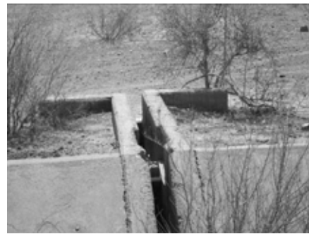
Tertiary canal diversion facility (Module Amasuk)
