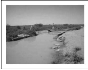
Upper stream of S27 secondary canal diversion
