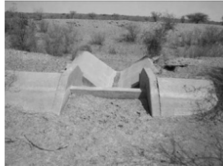
Secondary canal spillway
