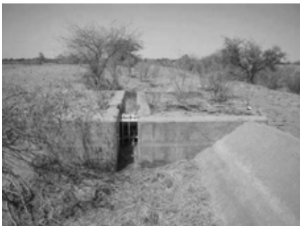
Tertiary canal diversion facility
