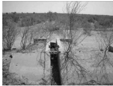
Tertiary canal diversion facility (Module Amasuk)
