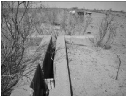
Tertiary canal diversion facility (Module Amasuk)
