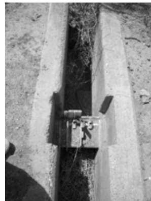
Tertiary canal diversion facility (Module Amasuk)
