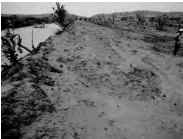
Reinforced dike (OA)
