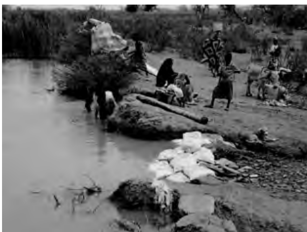
Reinforcement of dike with sandbags
