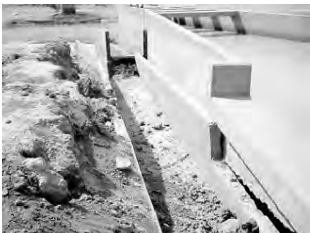
Damaged siphon
