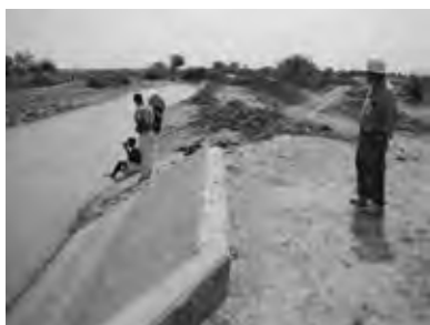
Strengthening of Dike at the Downstream of Aqueduct of Principal Canal AD
