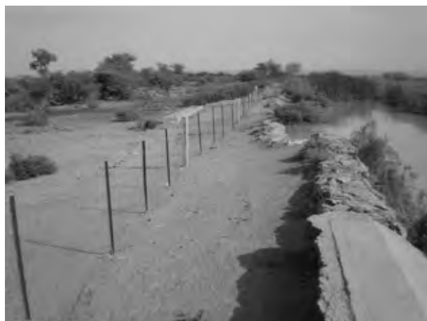
Protective fence against the Invasion of Livestock
