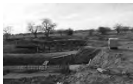
Bridge Construction on Road Between Kaedi and M'bout
