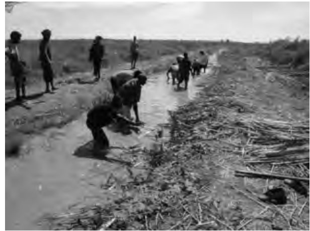
Dredging (Canal cleaning)
