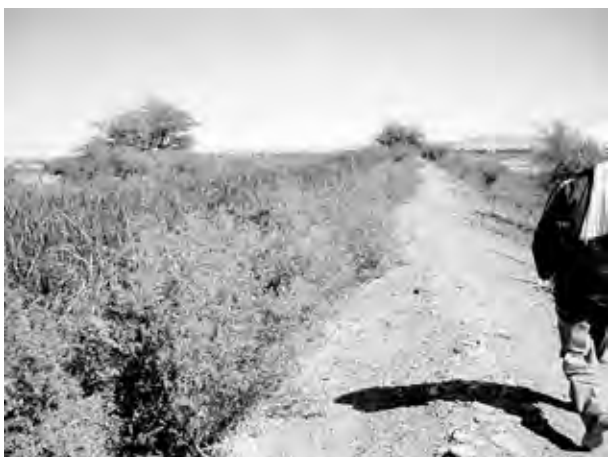
Main canal covered with Typha (AD)
