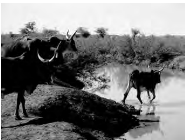
Damaged canal by livestock
