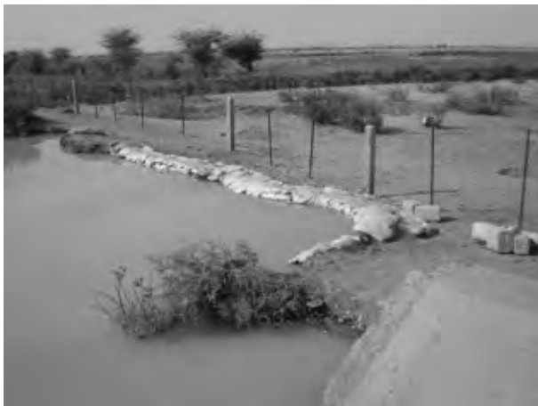
Strengthening by Sandbags S3
