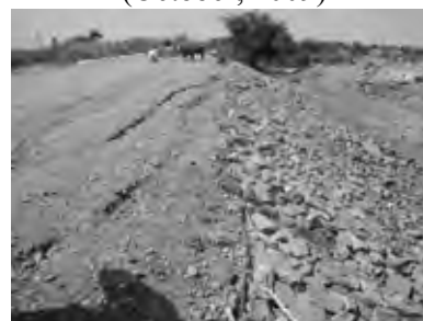
Strengthening of Dike at the Downstream of Aqueduct of Principal Canal AD
