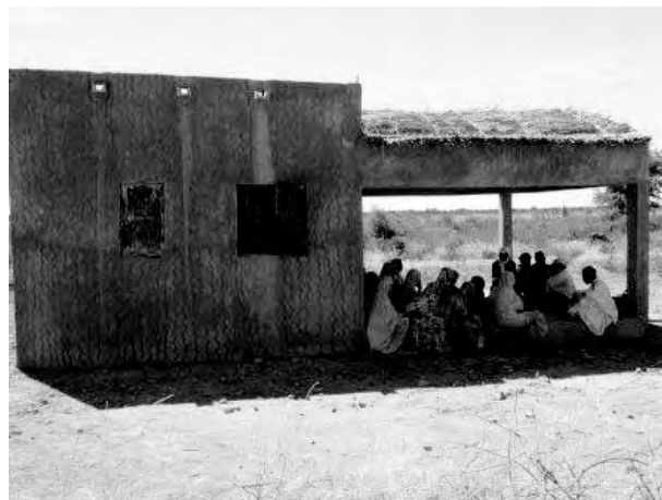
Establishment of multi-purpose shed
