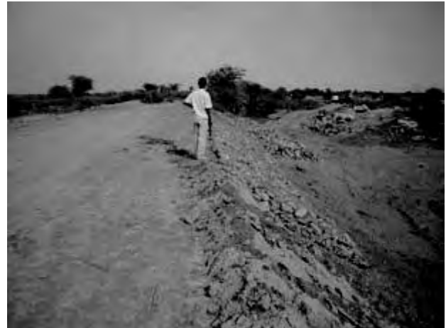
Embankment in downstream of bridge
