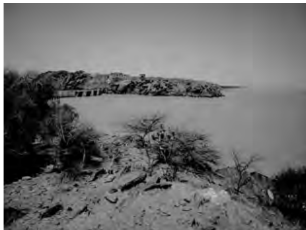
Dam and the reservoir
