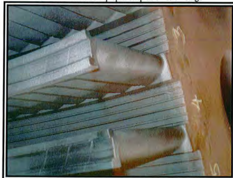
Photo - 19 IP – condition of Tip spill strip in 3 rd , 4 th & 5 th stage
