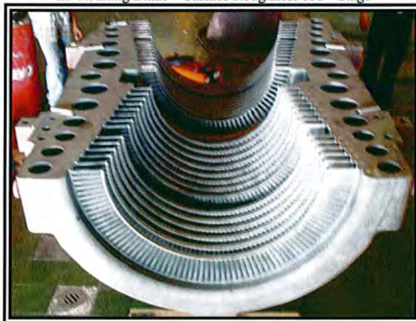
Photo 18 IP bottom Casing - after Sand Blasting
