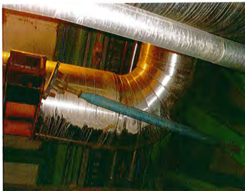
PHOTO 2- Dismantled Horz restraint in LPBP piping
