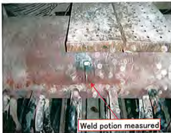
Measurement point of left side of RH outlet header
