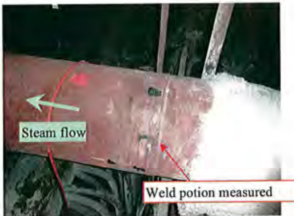
Measurement point of right De-superheater pipe
