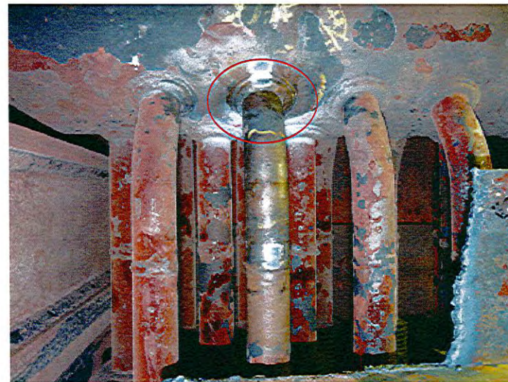
Example of inspection points
