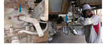
Fig. 6.13-2 Fly Ash Extraction Valve for Sampling
