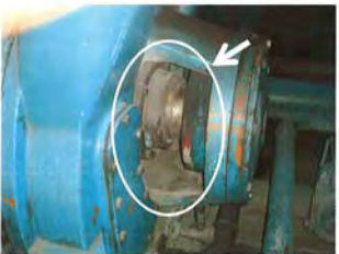
Photo-18: A-Vacuumpump grand seal (uncoupling side)
