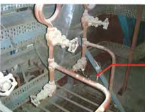
Photo-21 Injection test position (Drain pipe of Pressure transmitter for #6B vacuum pump inlet)
