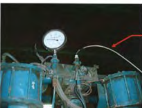
Photo-21 Injection test position (Drain pipe of Pressure transmitter for #6B vacuum pump inlet)
