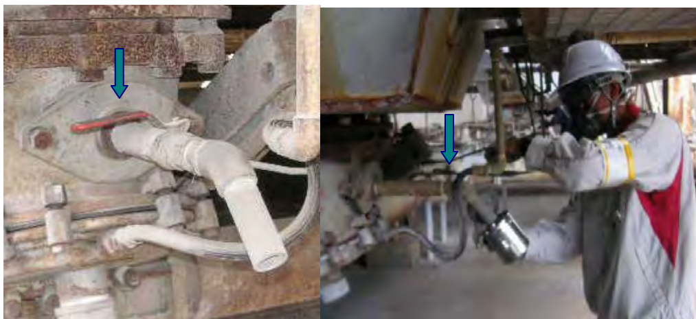
Fig. 6.13-2 Fly Ash Extraction Valve for Sampling
