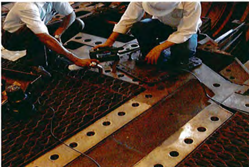
The view of MPI on parting plane of LP bottom casing.
