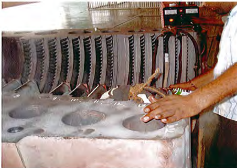
The view of Coil MPI testing on IP inner casing.
