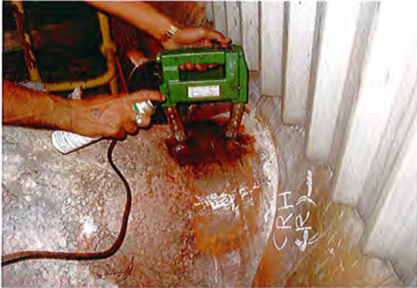
The MPI testing on weld joint of CRH line 9 th floor.
