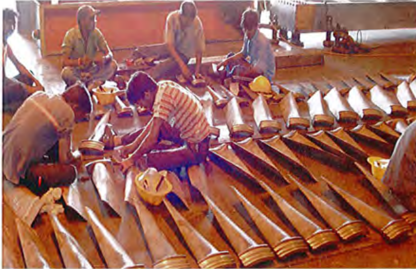
The view of cleaning of LP rotor blades.
