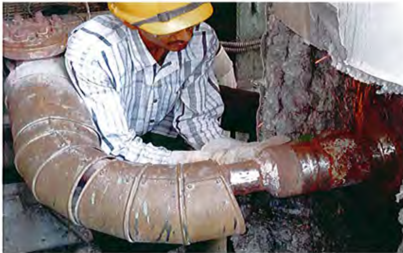
The cleaning of Scrub joint of HRH Line for testing.
