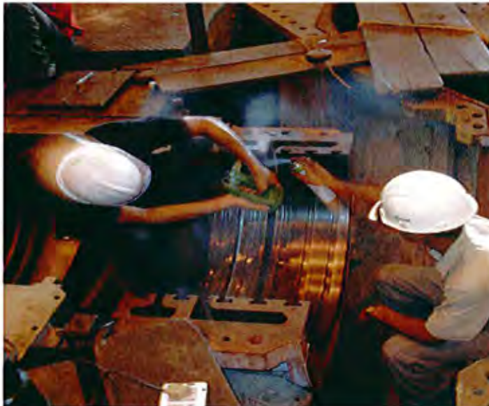
The view of MPI on bearing housing pedestal.
