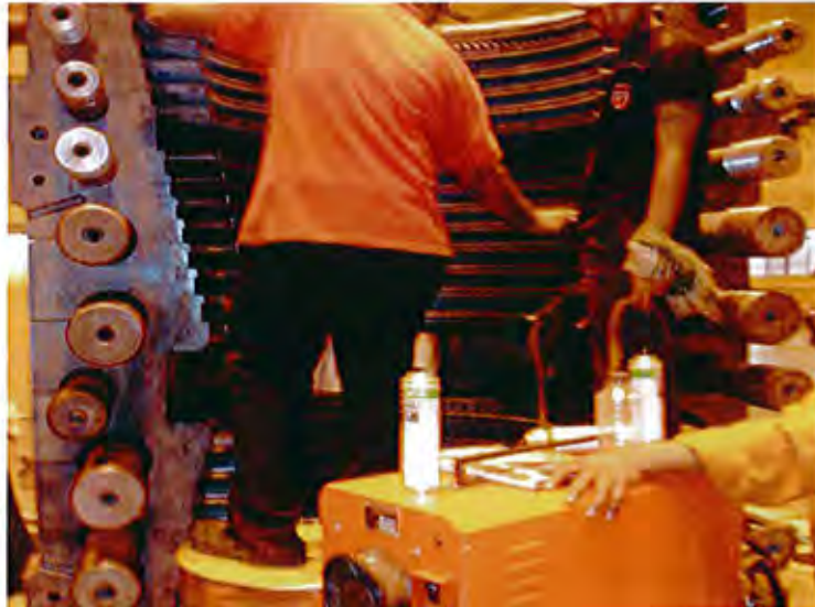
The view of Coil MPI testing on IP top inner casing.
