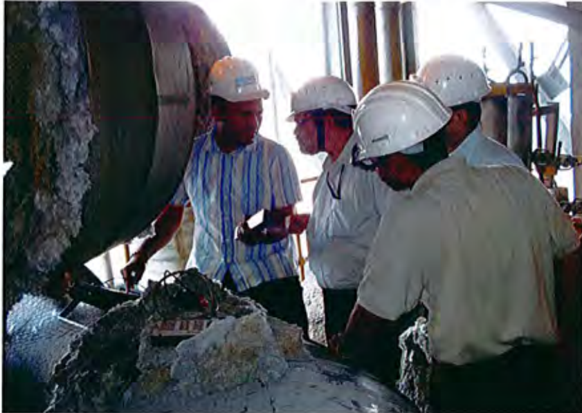
The view of UT testing on welding of HRH line.
