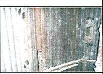
B: Erosion of Platen SH rear side tubes at the highest level of soot blower.
