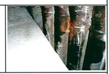
A: Erosion of water wall tubes near the corners.
