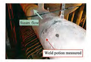
Measurement point of right De-superheater pipe
