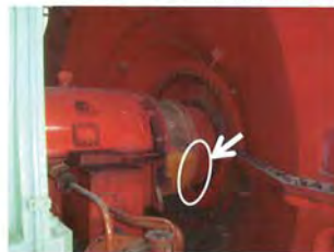
Photo-2: LP turbine packingland Turbine side (Upper/Left)
