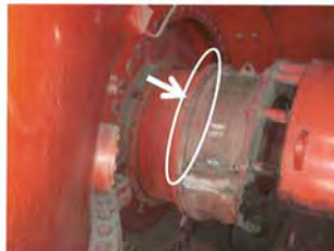
Photo-3: LP turbine packingland Turbine side (Lower/Left)
