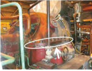
Photo-17: A-Vacuumpump grand seal (coupling side)
