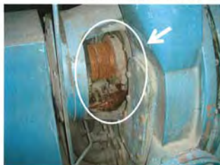
Photo-17: A-Vacuumpump grand seal (coupling side)
