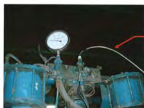
Photo-21 Injection test position (Drain pipe of Pressure transmitter for #6B vacuum pump inlet)
