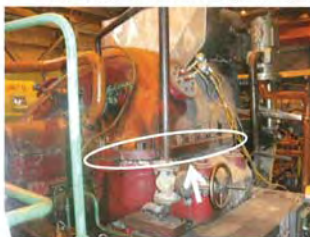
Photo-17: A-Vacuumpump grand seal (coupling side)
