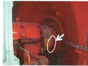
Photo-2: LP turbine packingland Turbine side (Upper/Left)
