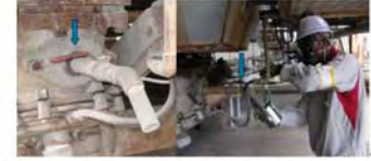
Fig. 6.13-2 Fly Ash Extraction Valve for Sampling 3)
