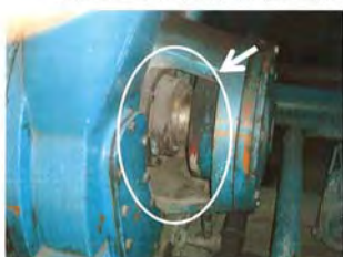
Photo-18: A-Vacuumpump grand seal (uncoupling side)
