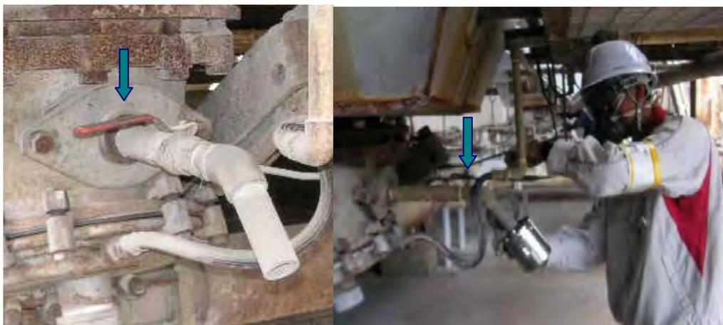
Fig. 6.13-2 Fly Ash Extraction Valve for Sampling
