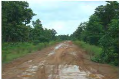
Bad Earth Section
