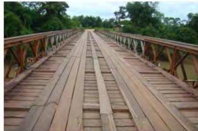
Long Bailey Bridge
