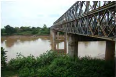
Long Bailey Bridge
