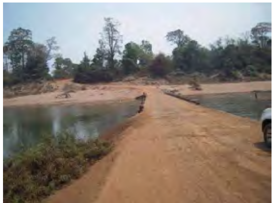
Existing Sedone Bridge (toward Salavan)
