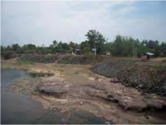
Gabion-mattress-based River bank protection around the bridge
