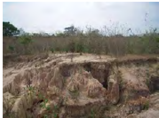
Large-scale roadside Erosion
